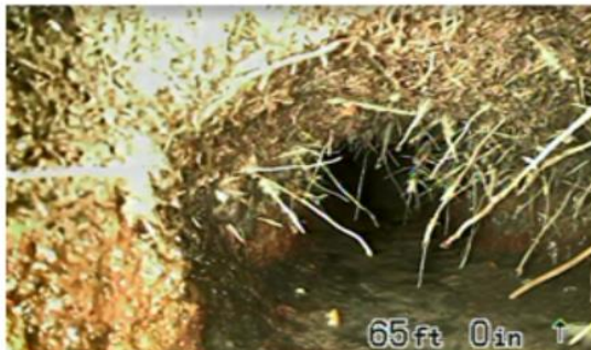
Defect C: Large offset with roots at 65 feet.
