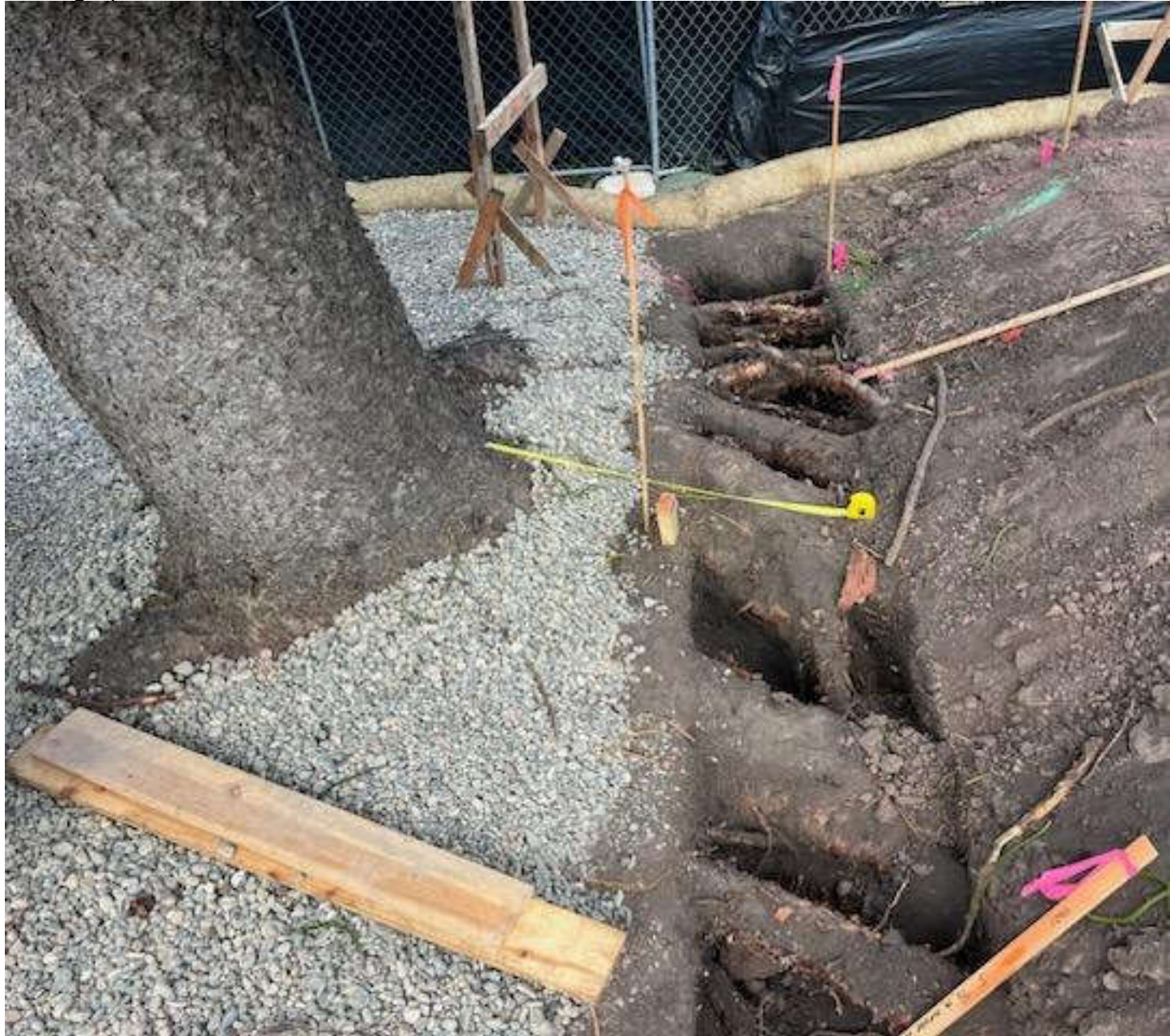
Photograph of Tree and Patio Foundation Trench
