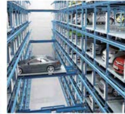
AUTOMATED PARKING CAN REDUCE SPACE PER CAR BY UP TO 50% WITH 2-3 MINUTE RETRIEVAL TIME
