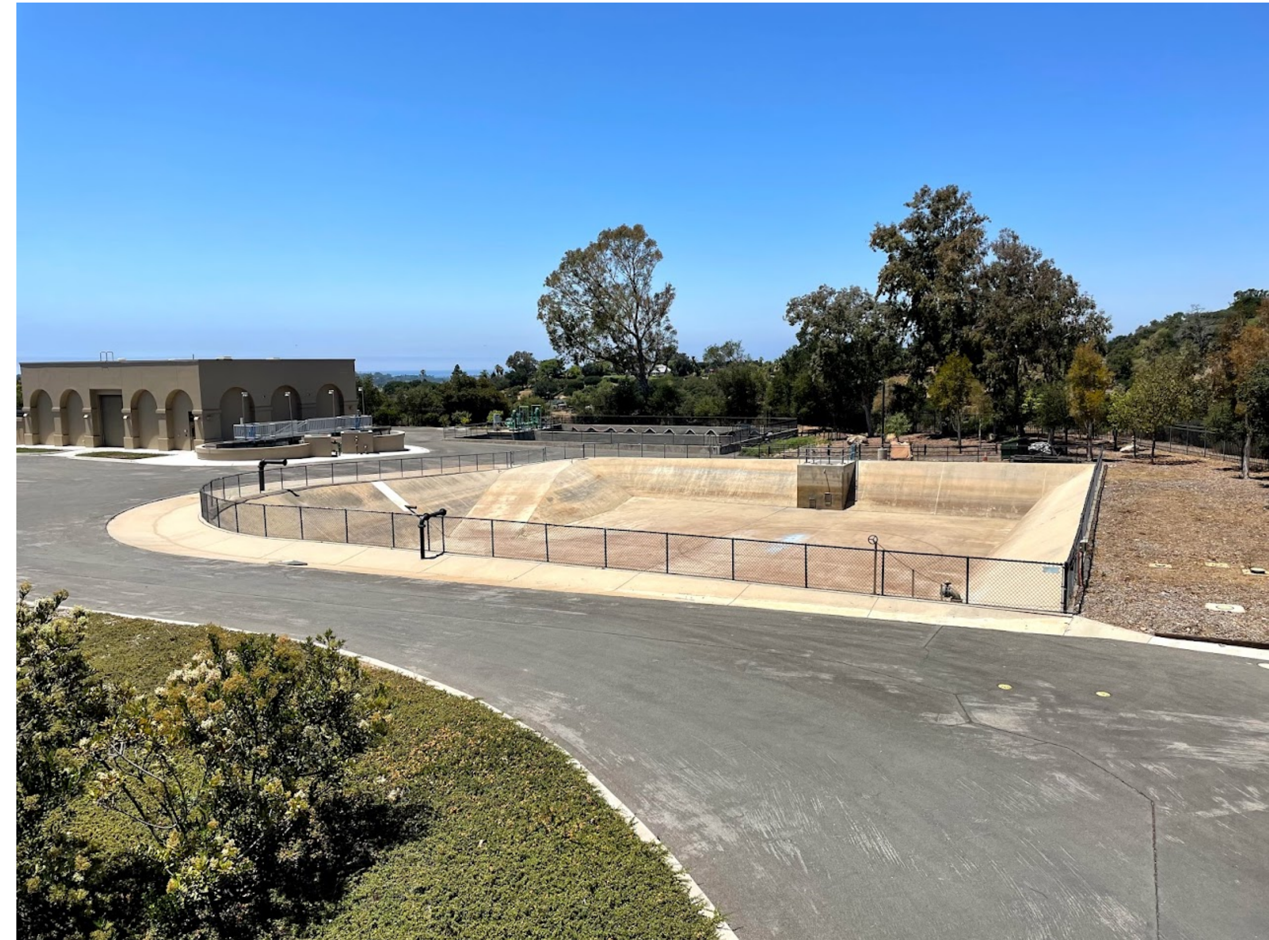
B 00GC01 EXISTING CONCRETE-LINED SLUDGE DRYING BED
