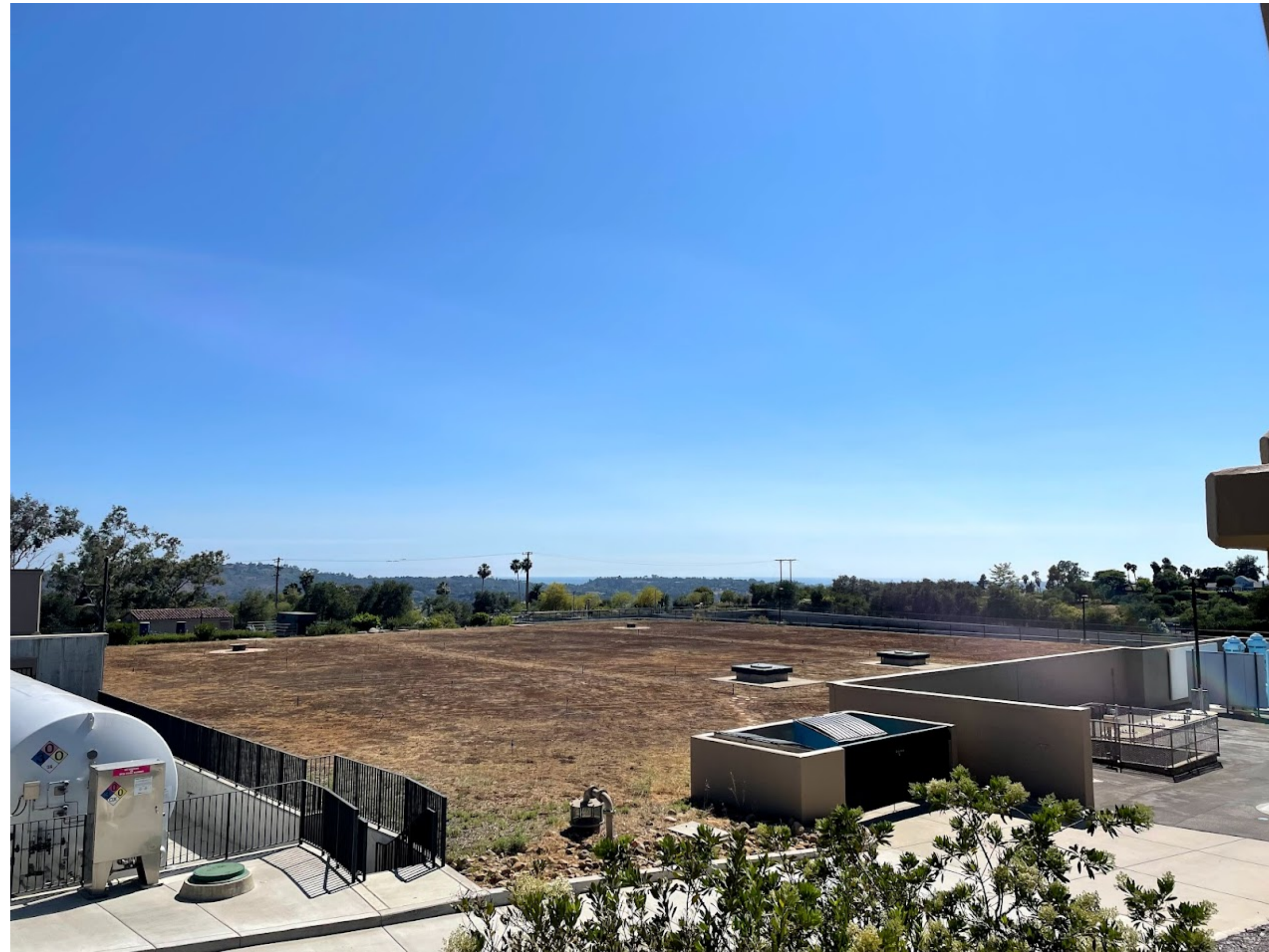
A 00GC01 EXISTING BURIED CLEARWELL
