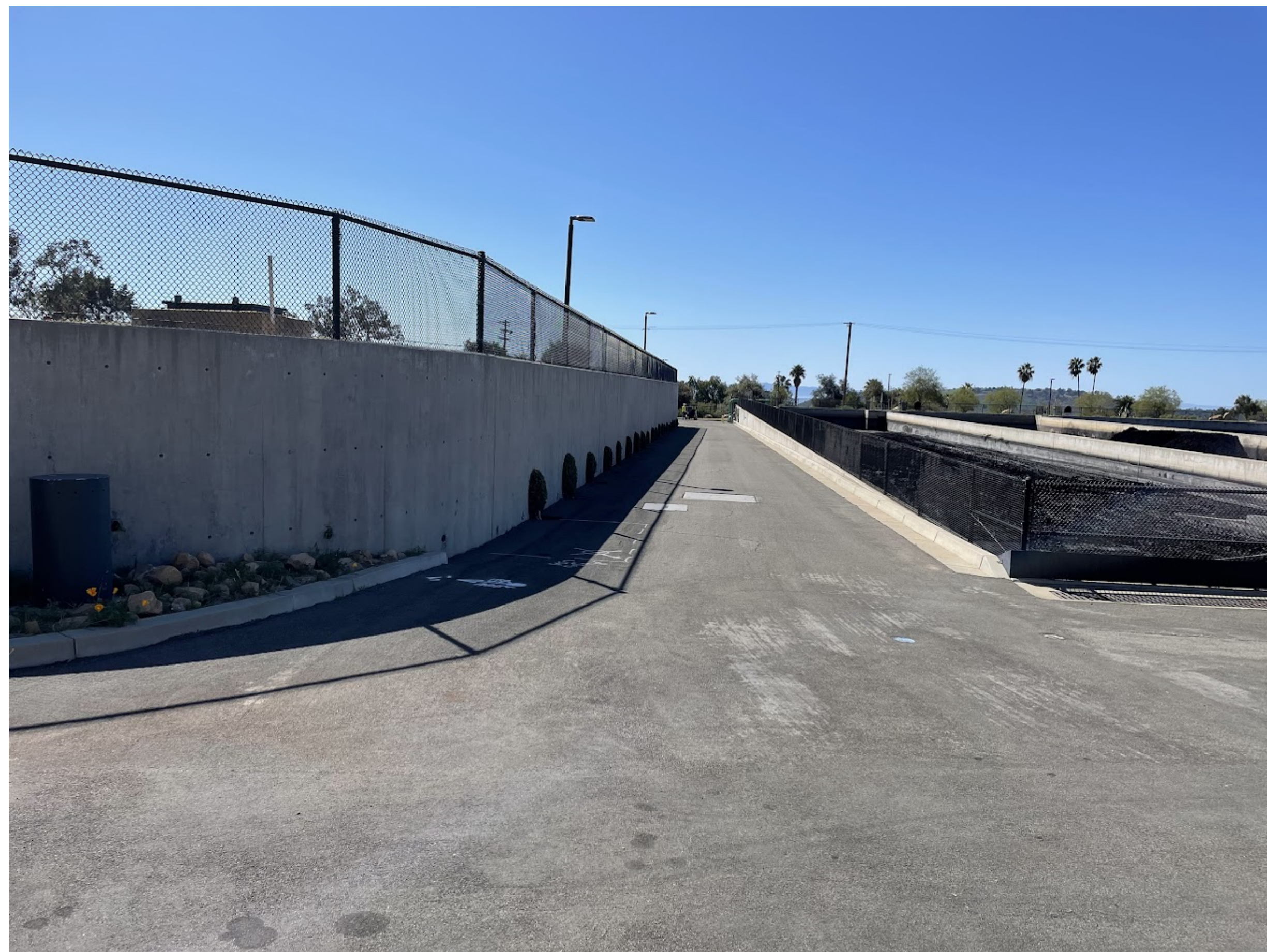
C 00GC01 EXISTING ROADWAY ADJACENT TO CLEARWELL (TO BE REMOVED)
