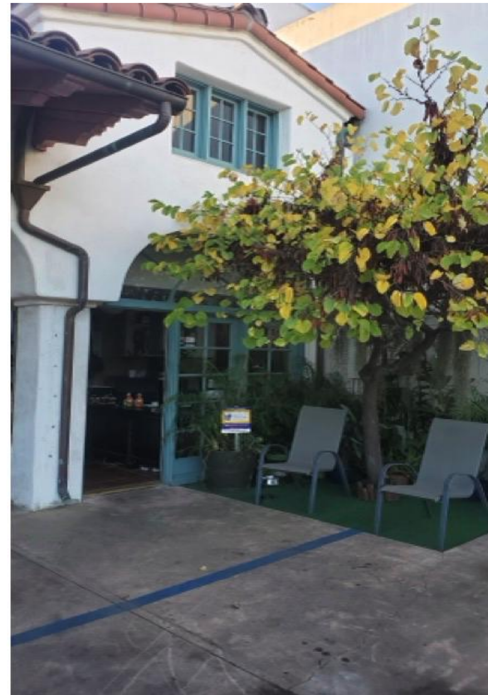
7 APPROACHING NORTH ELEVATION FROM PARKING LOT
