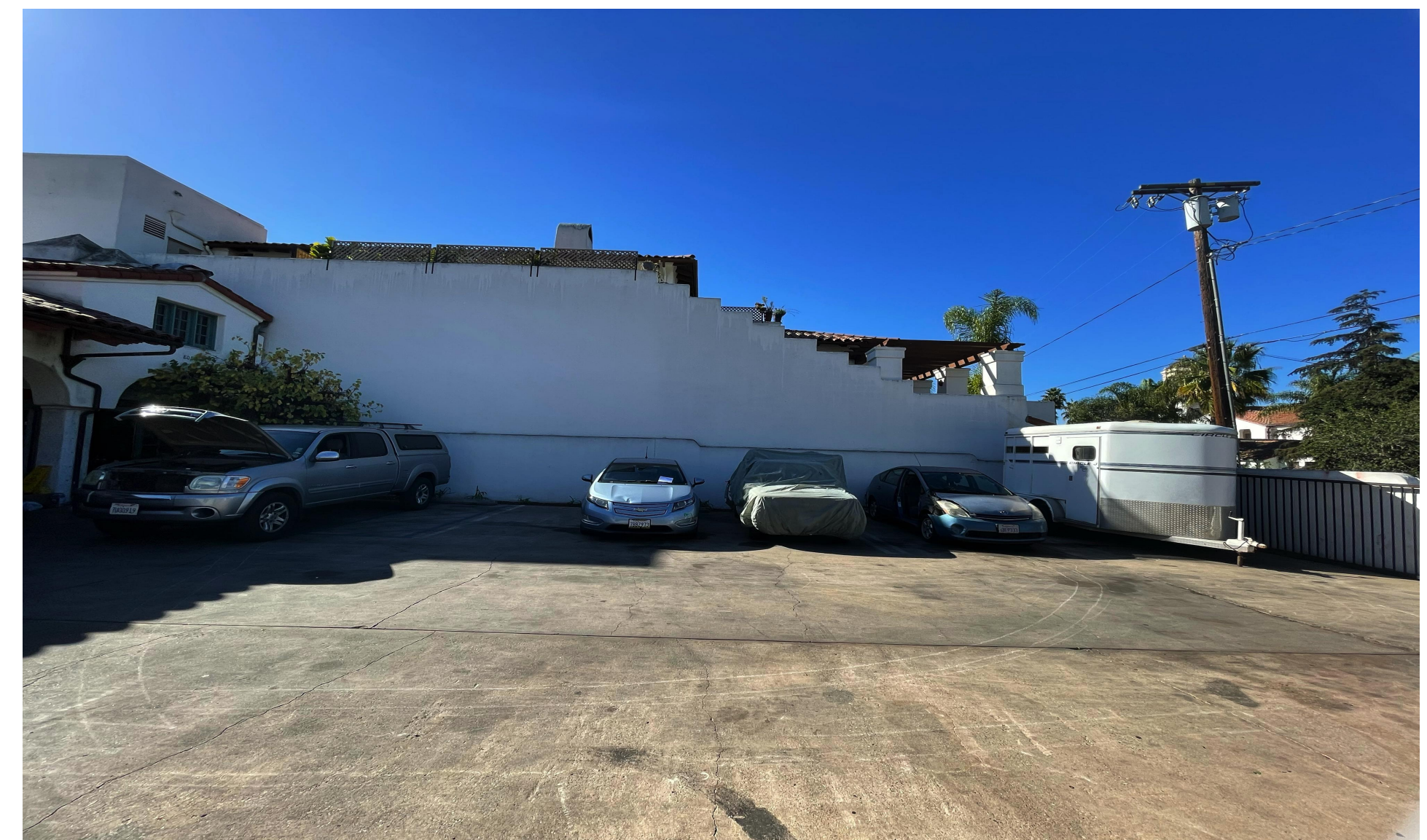
1 LOOKING AT WEST ELEVATION FROM PARKING LOT
