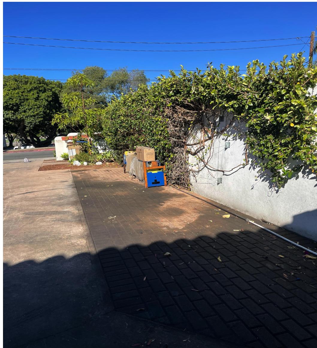
11 LOOKING AT EAST ELEVATION FROM PARKING LOT
