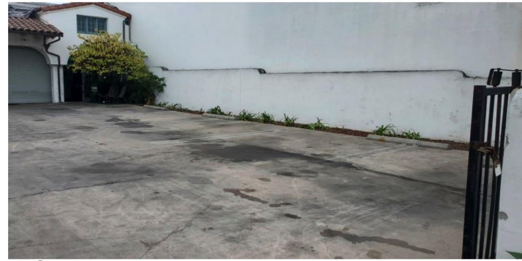
2 LOOKING AT WEST ELEVATION FROM COTA STREET SIDE WALK
