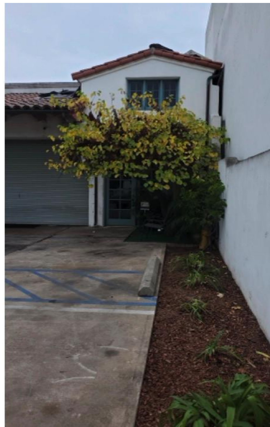
6 APPROACHING NORTH ELEVATION FROM PARKING LOT
