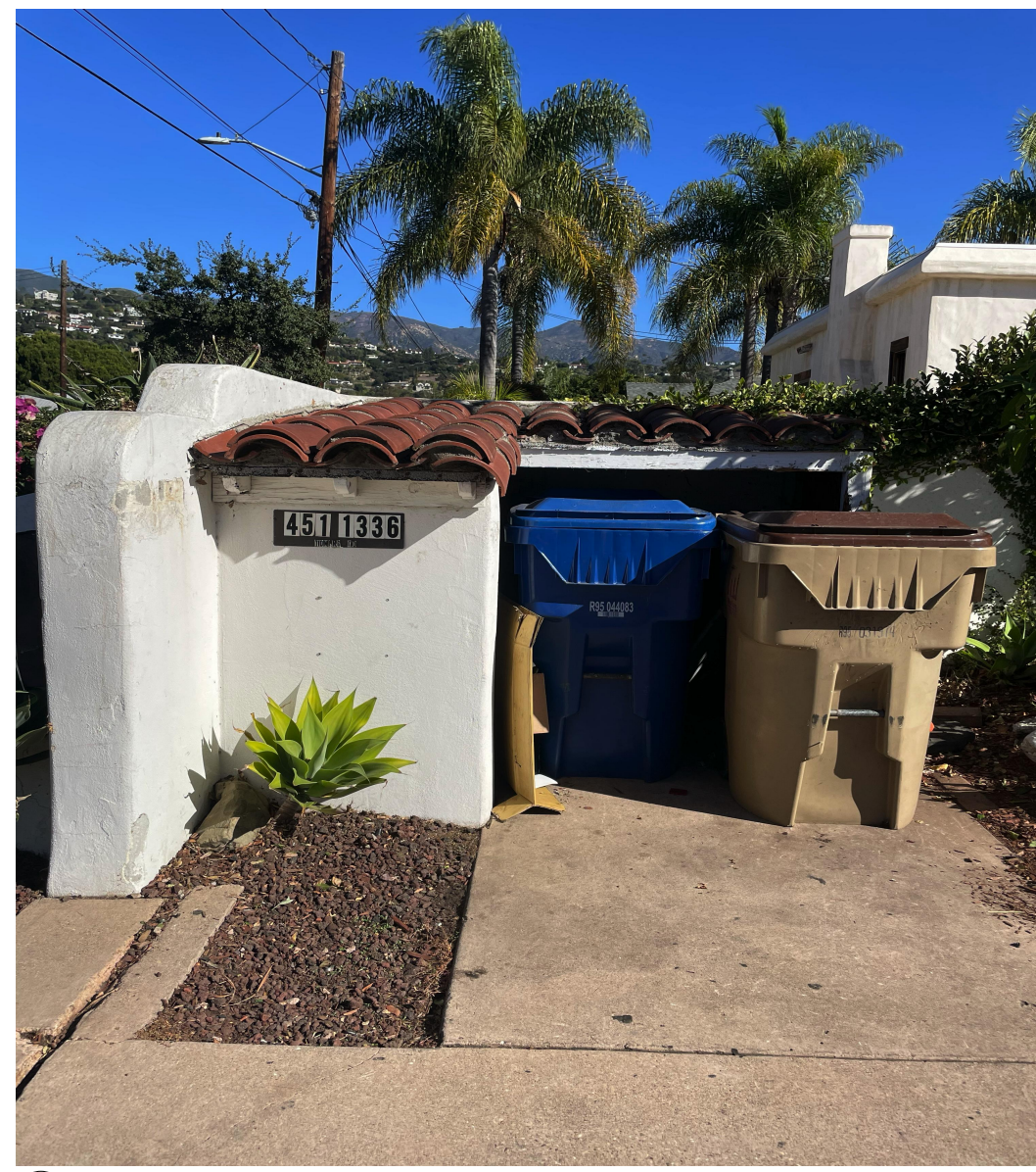
9 APPROACHING TRASH ENCLOSURE FROM PARKING LOT
