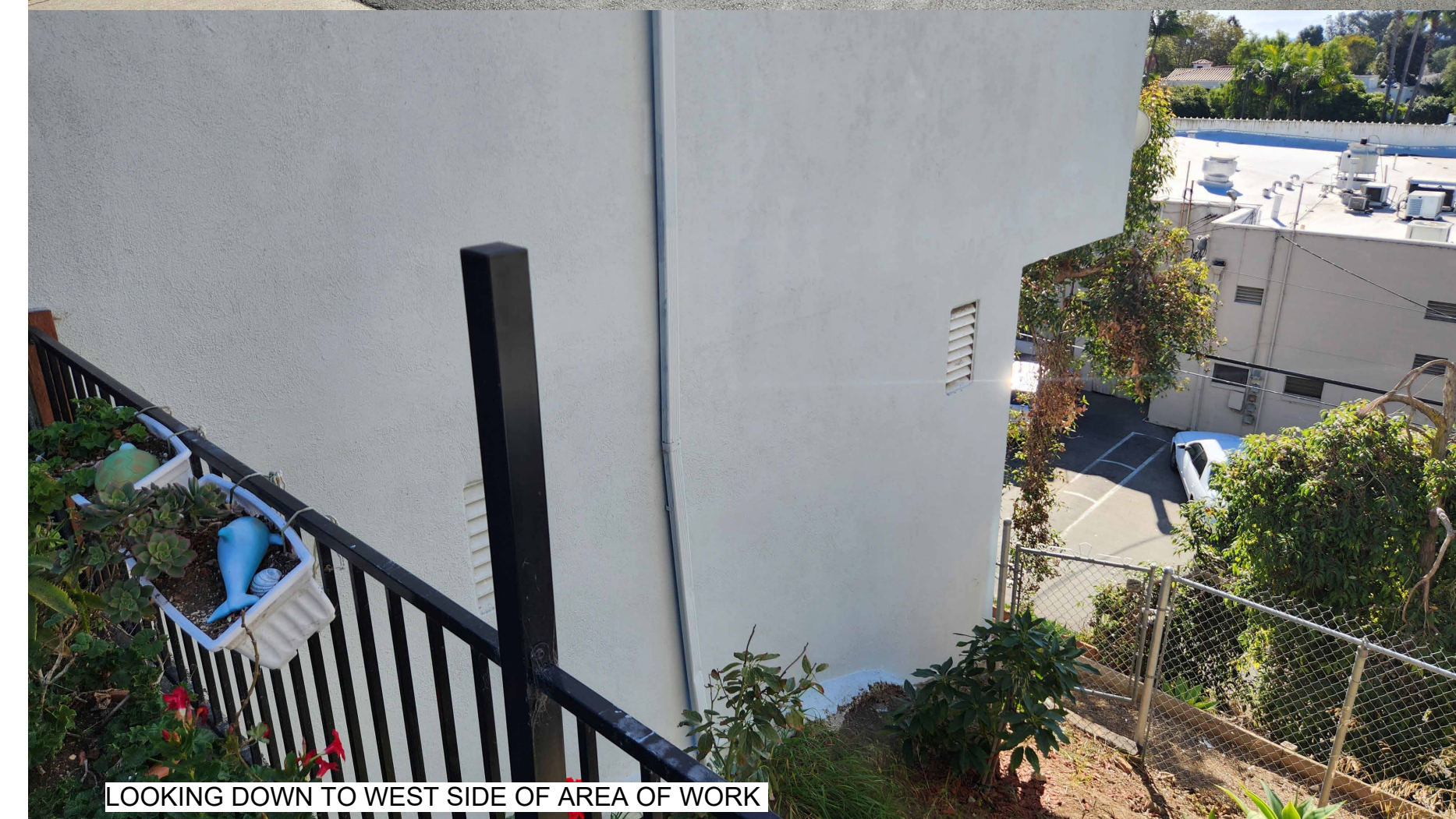
LOOKING DOWN TO WEST SIDE OF AREA OF WORK
