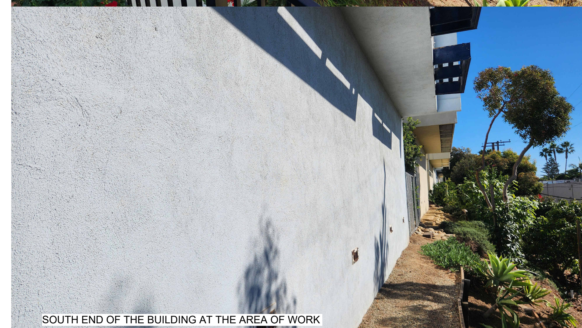
SOUTH END OF THE BUILDING AT THE AREA OF WORK
