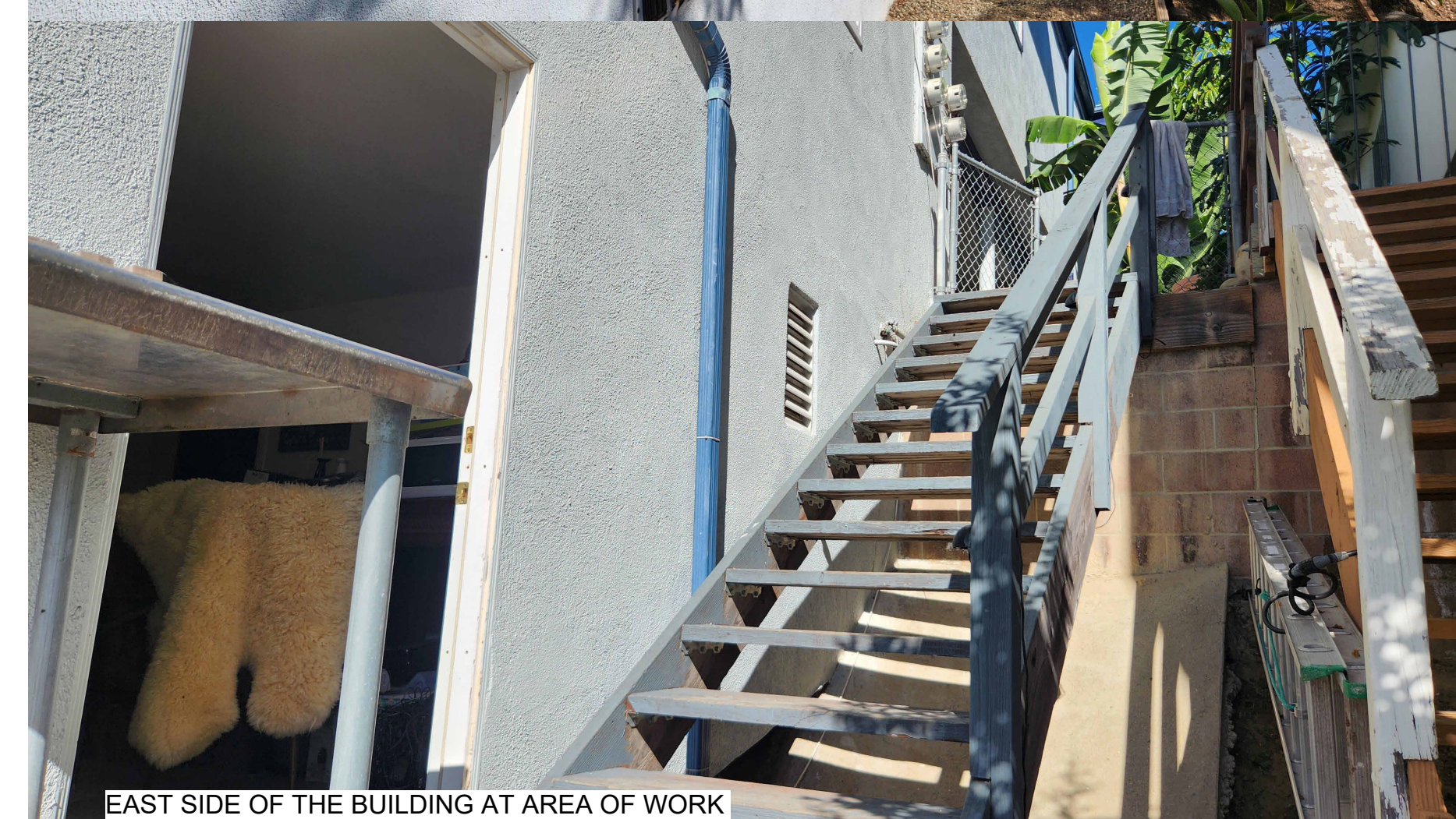
EAST SIDE OF THE BUILDING AT AREA OF WORK
