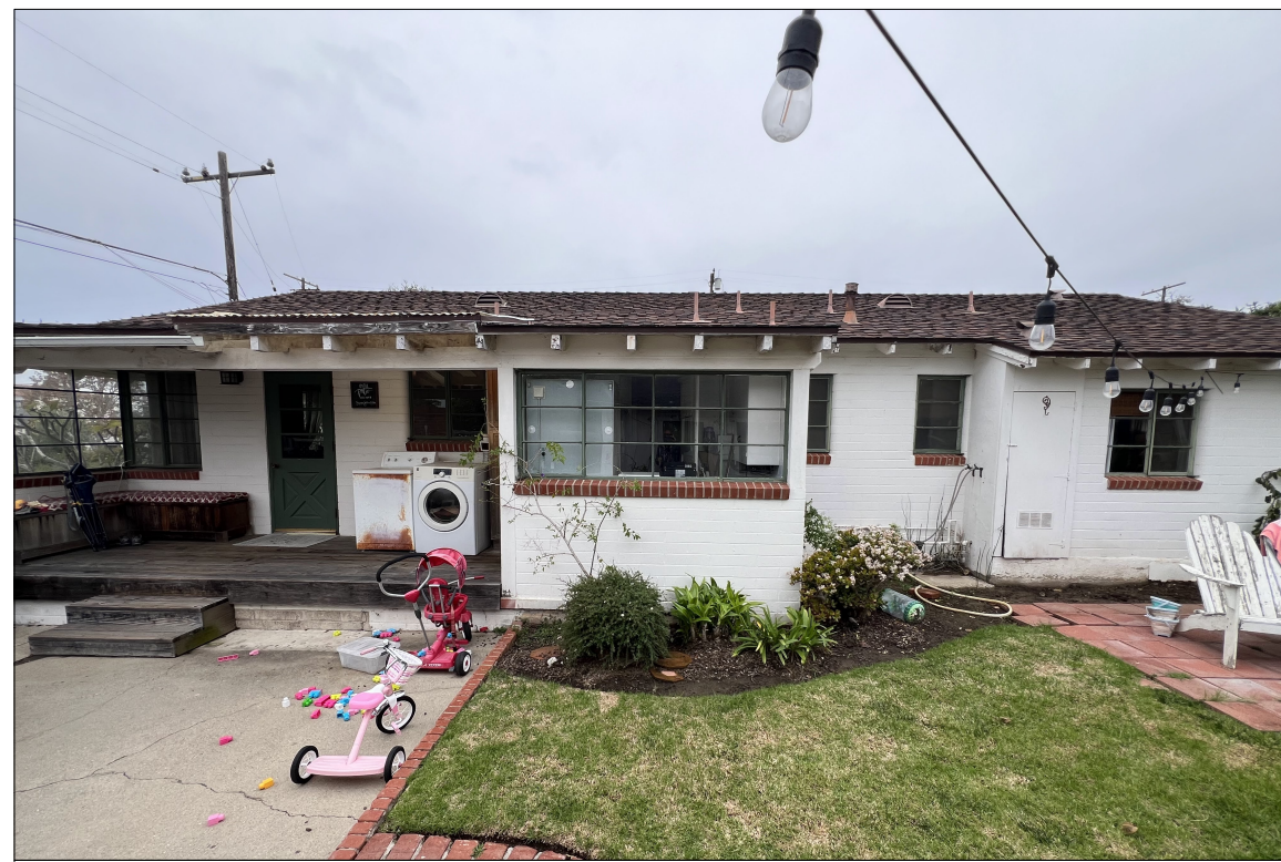
#3 - LOOKING WEST @ PROJECT SITE (PRIMARY DWELLING)
