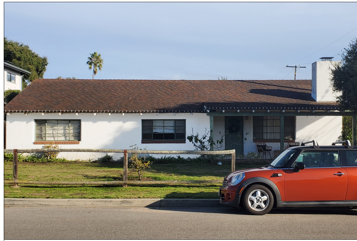
#1 - LOOKING EAST @ PROJECT SITE (PRIMARY DWELLING)
