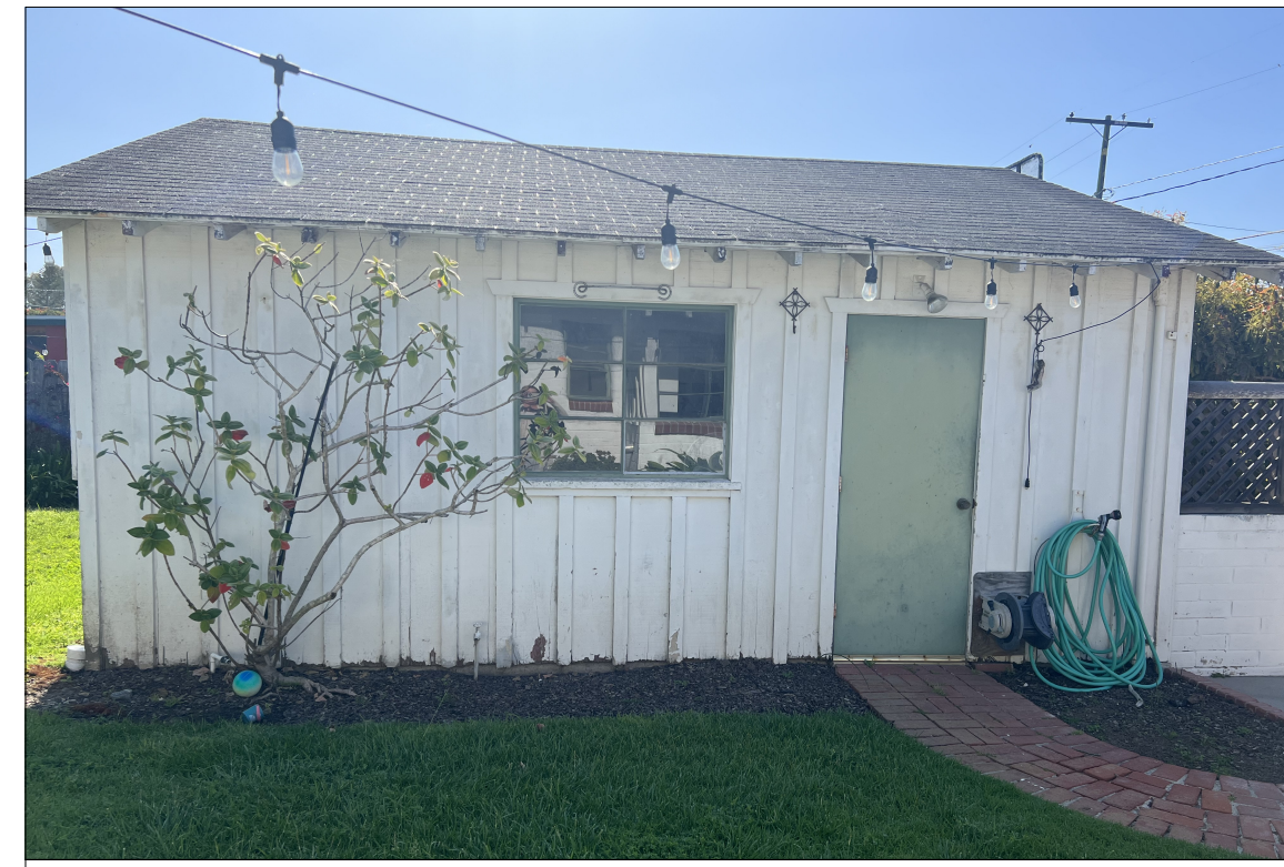
#6 - LOOKING EAST @ PROJECT SITE (DETACHED GARAGE)
