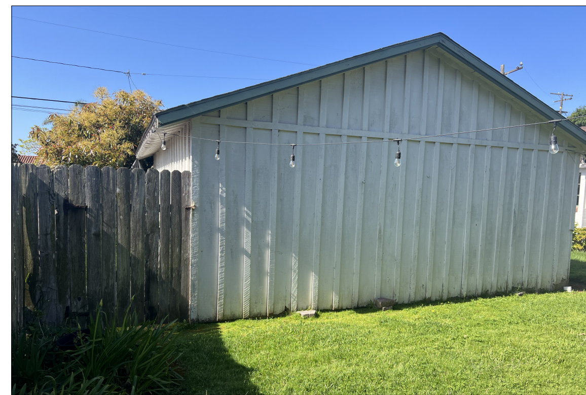
#8 - LOOKING WEST @ PROJECT SITE (DETACHED GARAGE)
