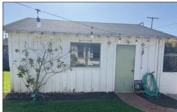
#6 - LOOKING EAST @ PROJECT SITE (DETACHED GARAGE)
