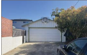
#5 - LOOKING NORTH @ PROJECT SITE (DETACHED GARAGE)
