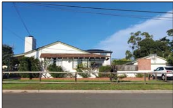
#2 - LOOKING NORTH @ PROJECT SITE (PRIMARY DWELLING)
