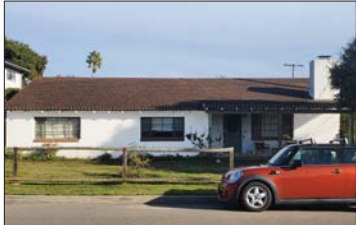
#1 - LOOKING EAST @ PROJECT SITE (PRIMARY DWELLING)
