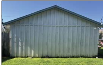
#7 - LOOKING NORTH @ PROJECT SITE (DETACHED GARAGE)
