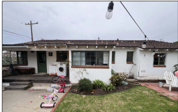
#3 - LOOKING WEST @ PROJECT SITE (PRIMARY DWELLING)
