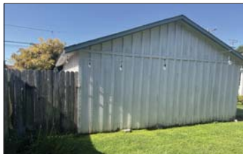
#8 - LOOKING WEST @ PROJECT SITE (DETACHED GARAGE)
