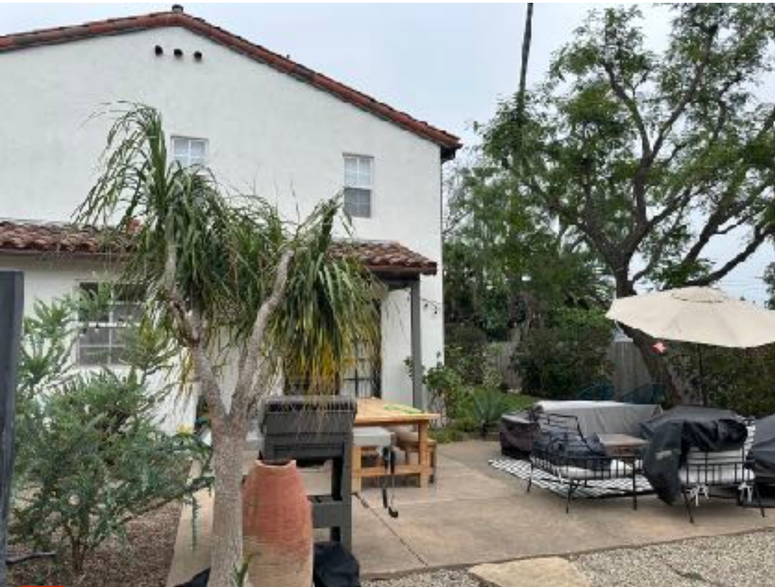
7 SIDE OF HOUSE FROM POOL AREA - FACING EAST
