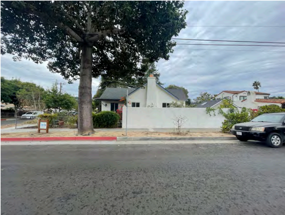
FACING 902 W. ISLAY STREET FROM GILLESPIE STREET (PRIMARY RESIDENCE)
