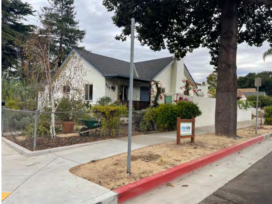
FACING 902 W. ISLAY STREET FROM THE INTERSECTION OF W. ISLAY STREET & GILLESPIE STREET (PRIMARY RESIDENCE)
