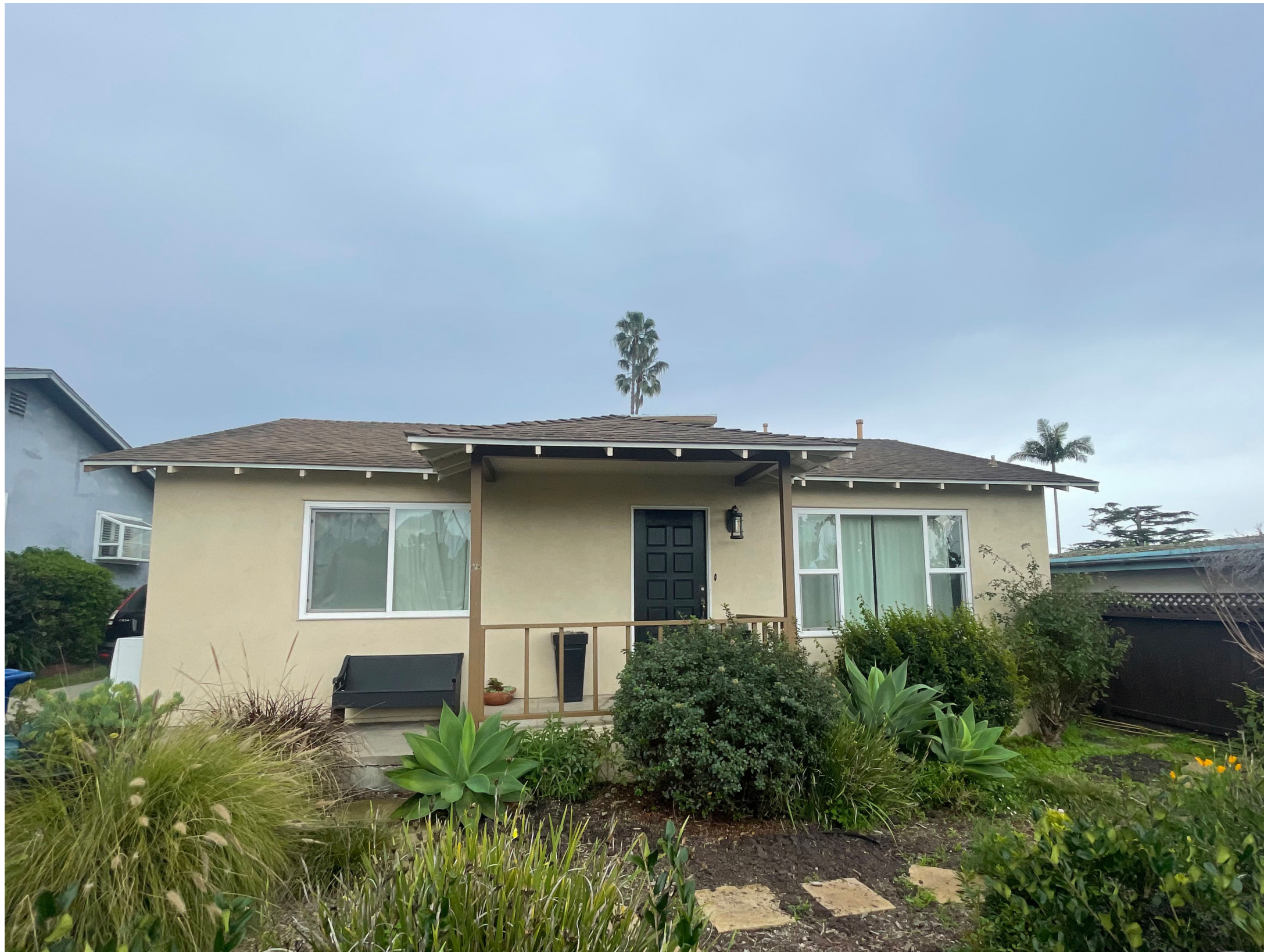
1) 412 Flora Vista - From Street (From West looking East)
