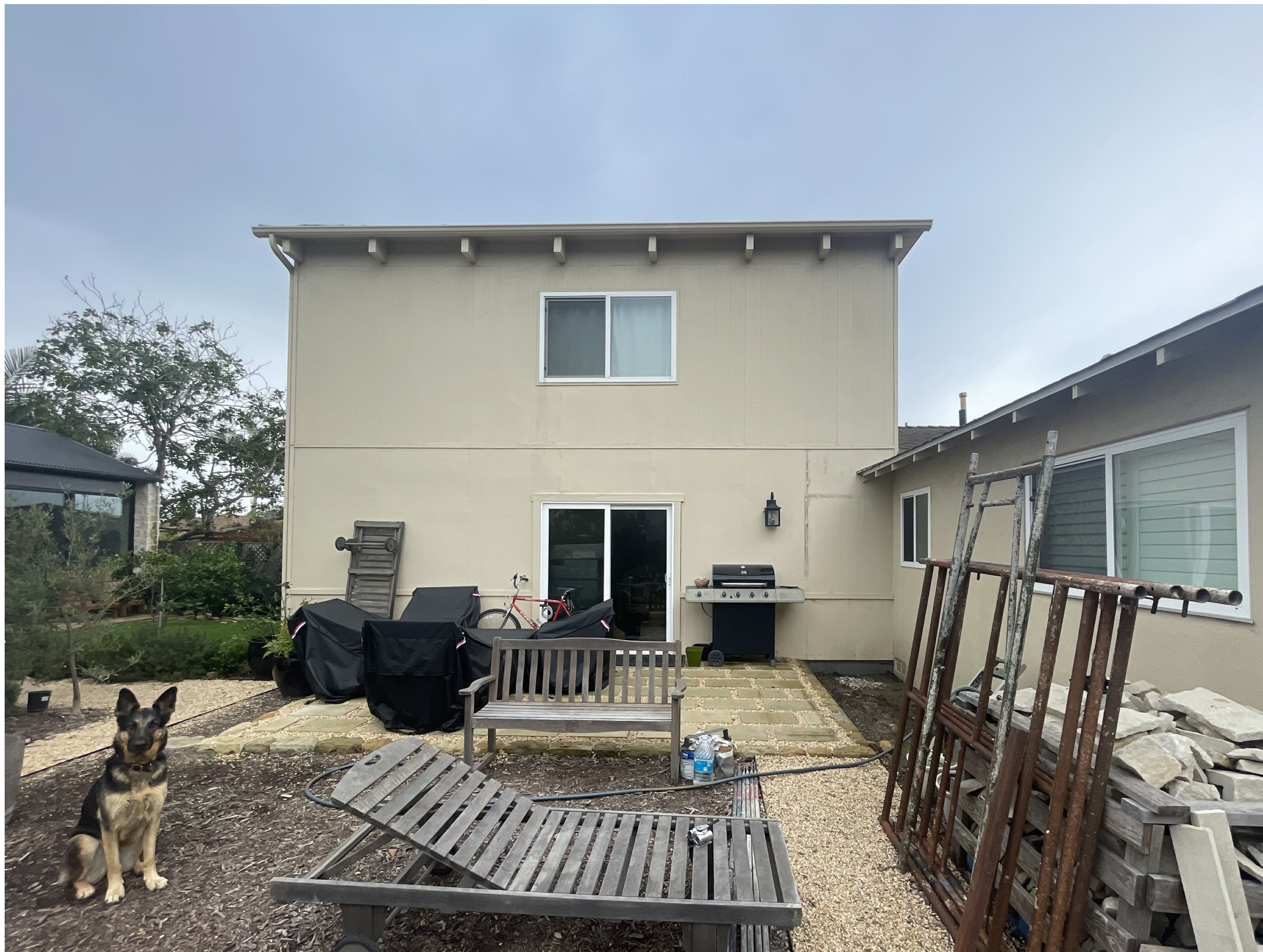
3) 412 Flora Vista - From North looking South
