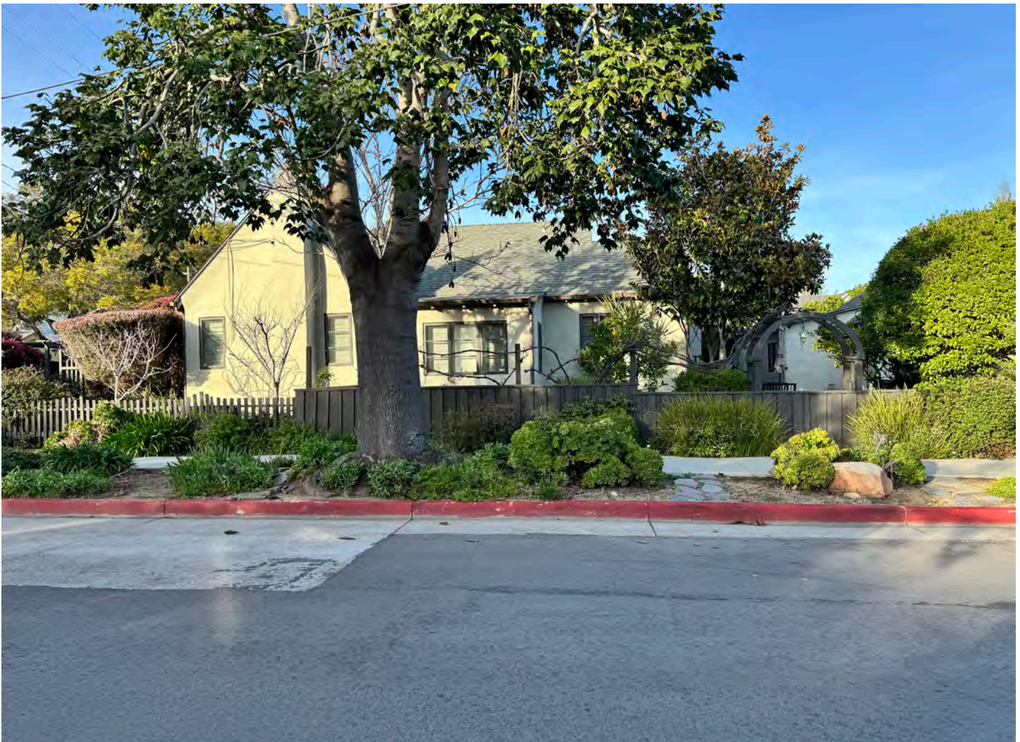
1 - LOOKING NORTH EAST
