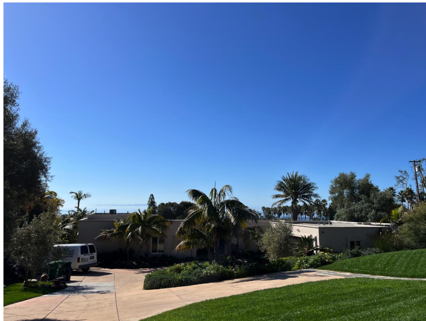
LOOKING SOUTH FROM DRIVEWAY TOWARDS MAIN RESIDENCE AND AREA OF ALTERATION
