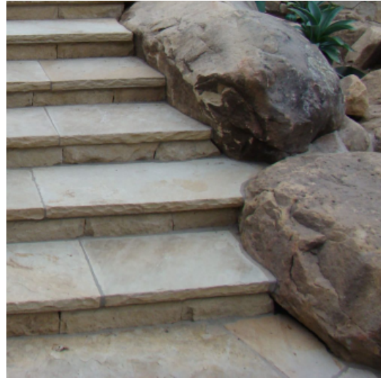
STONE STEPS INTERFACE WITH BOULDERS
