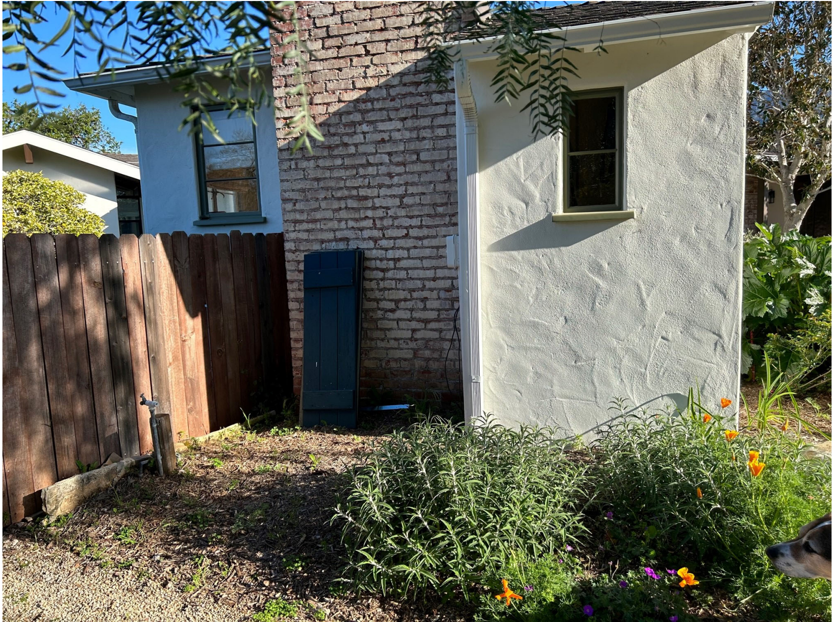
Photo 9 – South Elevation of Subject Property
