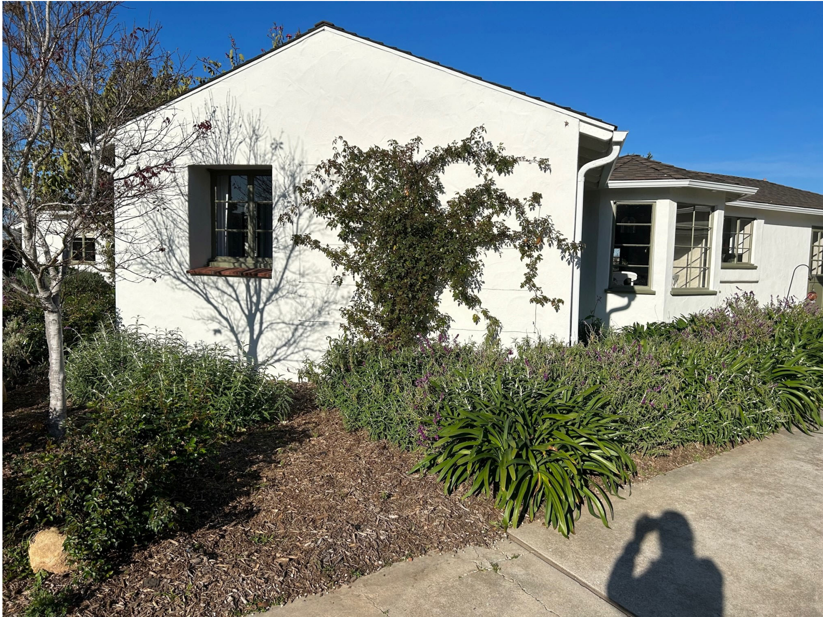
Photo 8 – East Elevation of Subject Property
