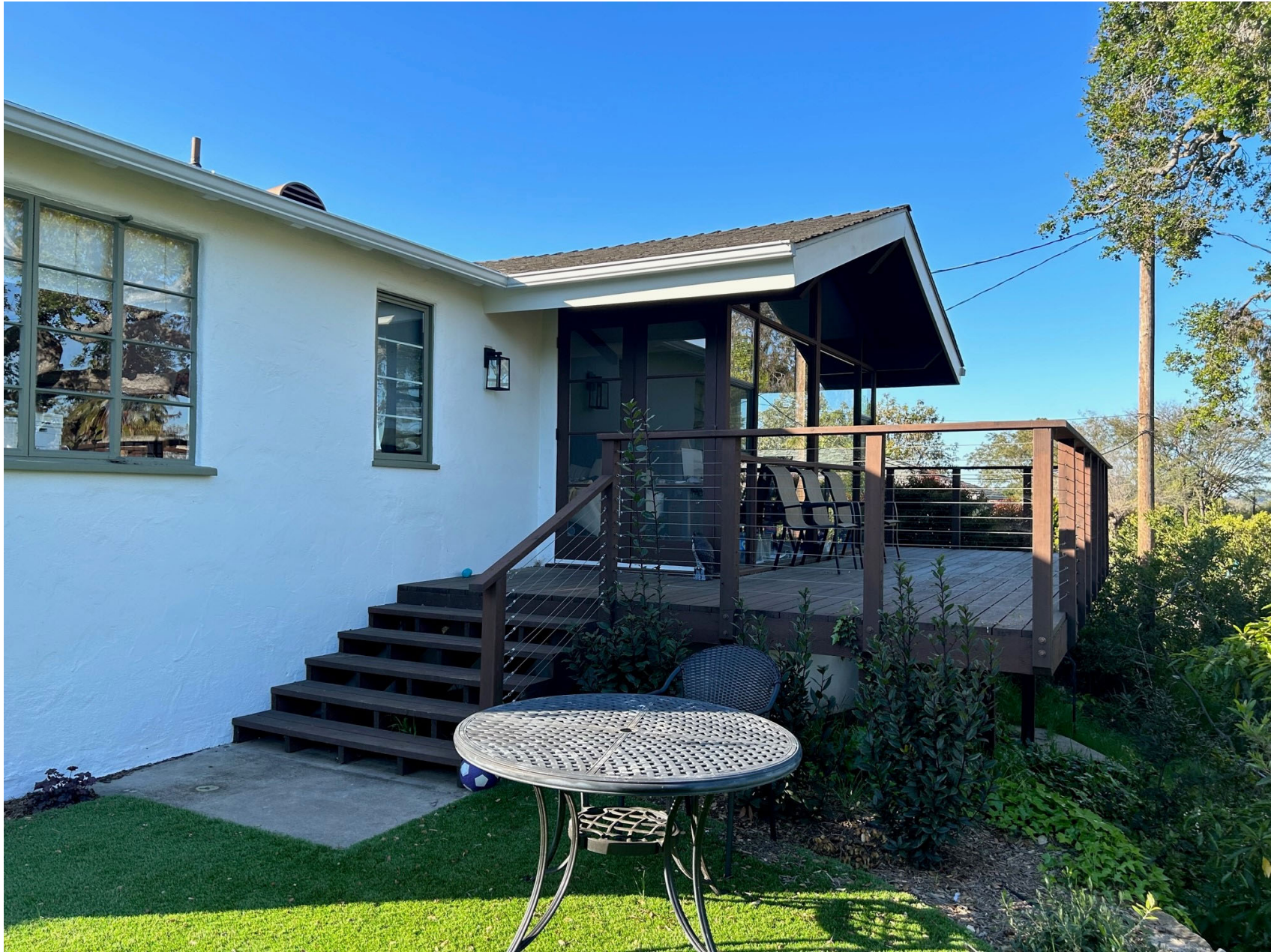
Photo 7 – Northwest view of Subject Property
