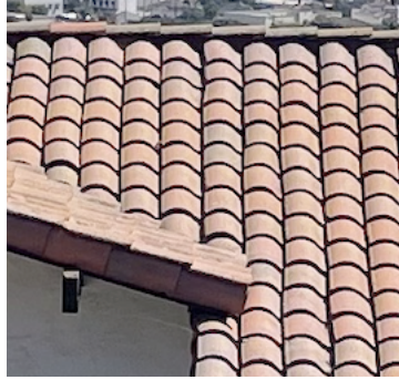
SPANISH TILE TILE 1: CLAY TILE TO MATCH (E) REDLANDS ALFARO 3010 "TERRA COTTA BLEND"
