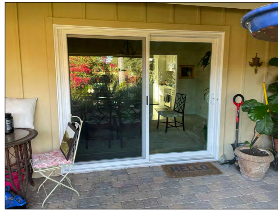
#5: EAST ELEVATION (LIVING ROOM DOORS)
