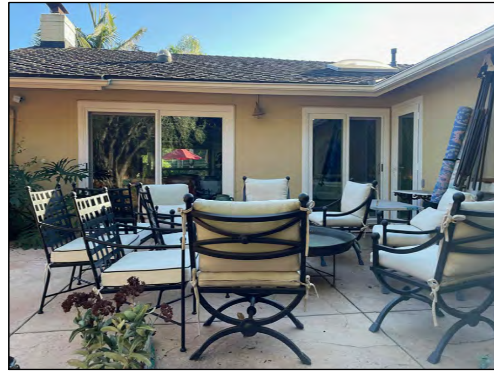
#7: NORTH ELEVATION (LIVING & BEDROOM DOORS)
