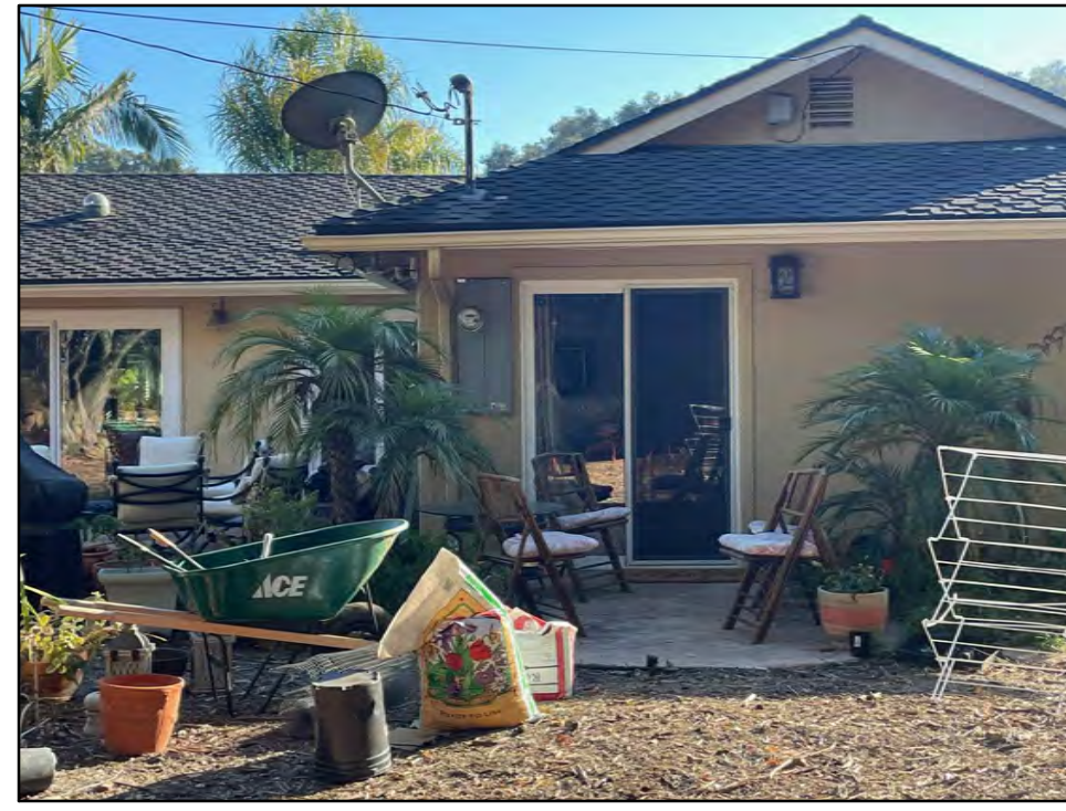
#8: NORTH ELEVATION (MASTER BEDROOM DOOR)
