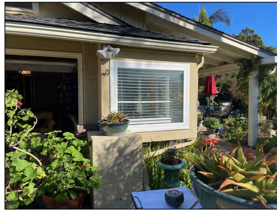
#4: GARAGE #1 CORNER WINDOW
