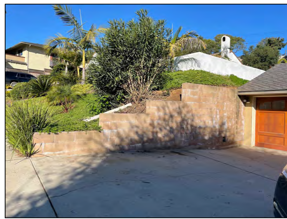
#1: RETAINING WALL AND GARAGE #2
