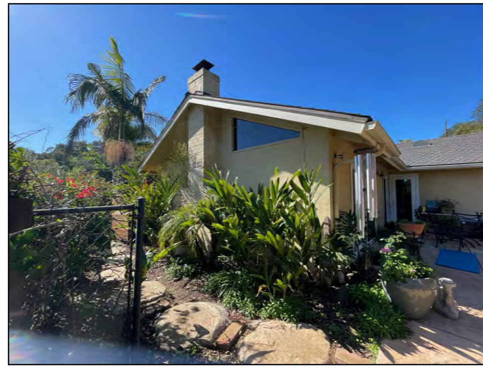
#6: EAST ELEVATION (LIVING ROOM CLERESTORY WINDOWS)
