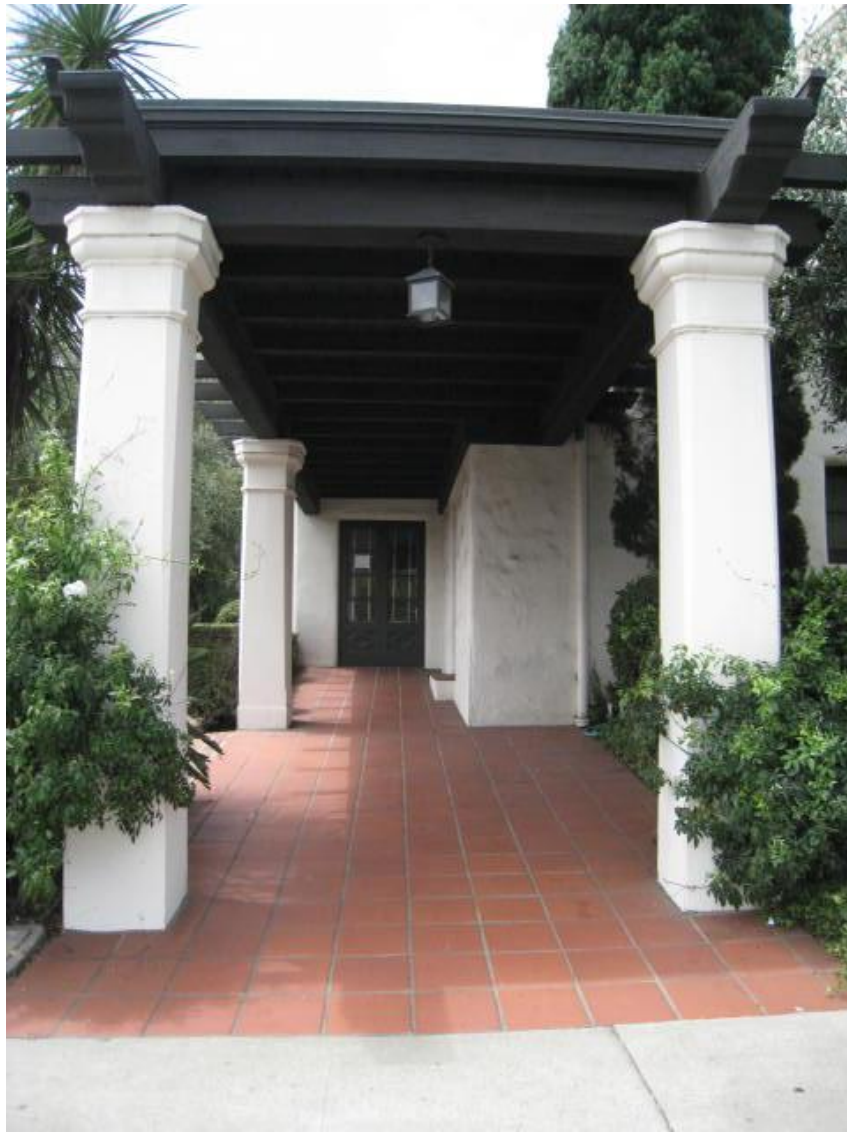
Plate 10. East elevation of pergola at Anacapa Street where steps will be added. Facing east.
