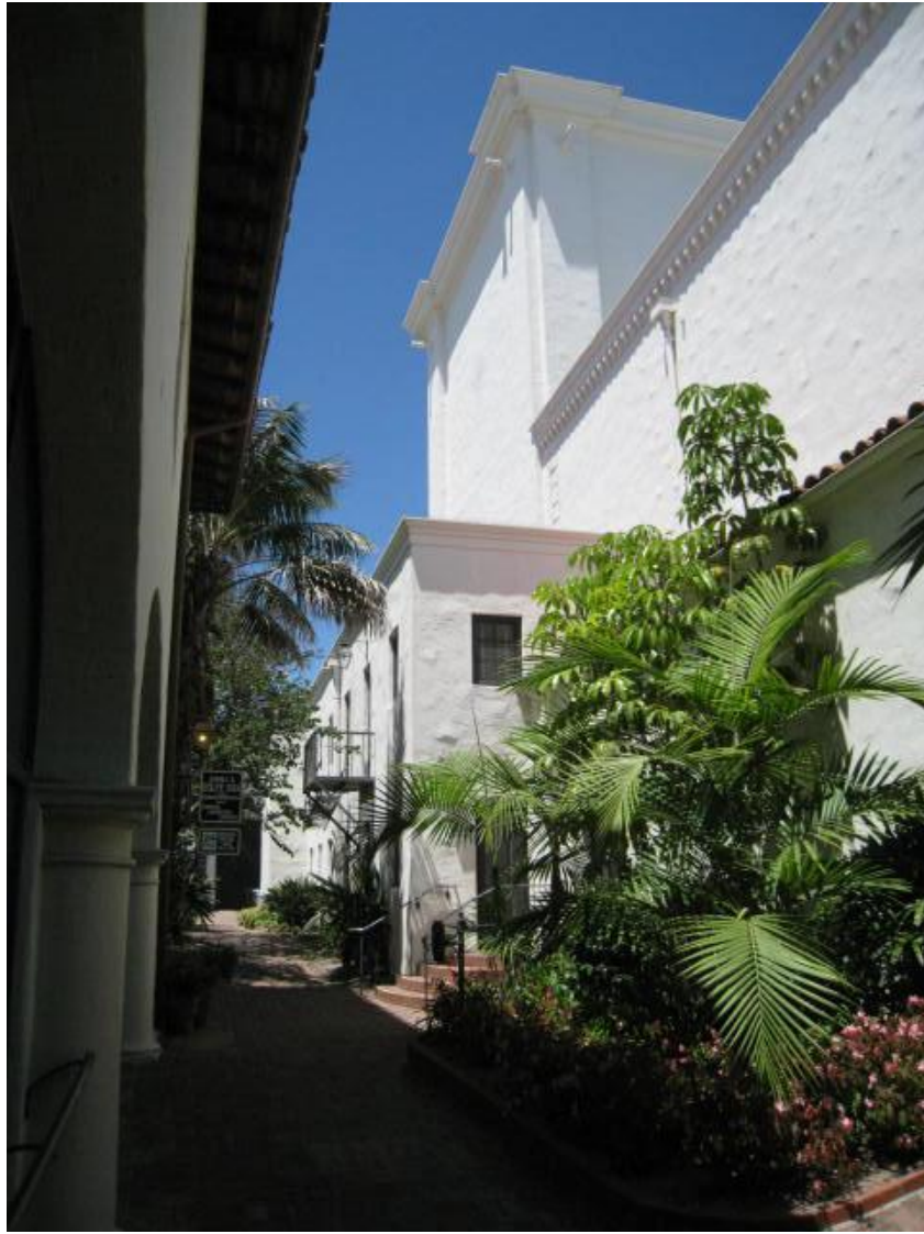
Plate 6. View from west pathway showing Green Room roof where added HVAC equipment will be hidden by high wall. Facing north.
