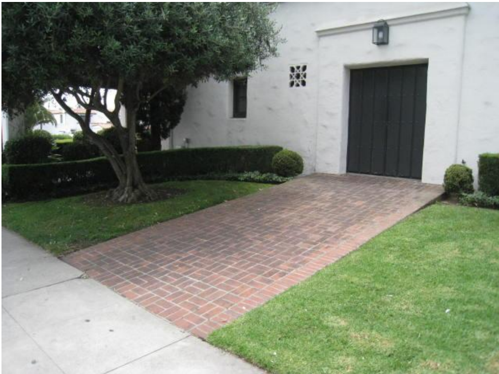
Plate 8. East exit door where steps will be added. Facing southwest.
