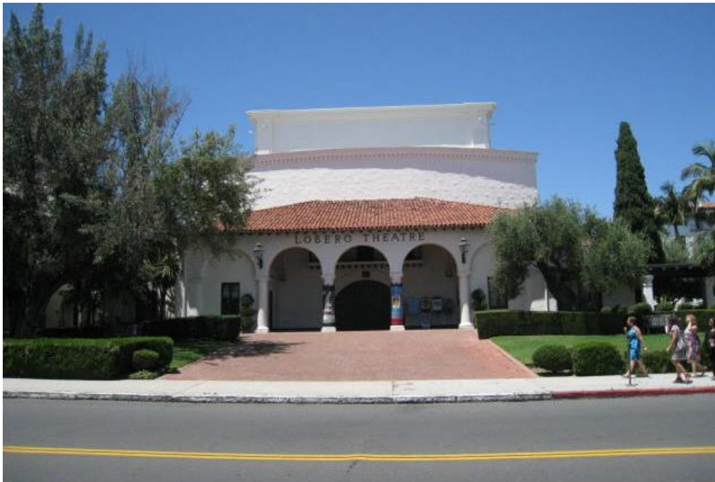
Plate 1. South elevation showing brick ramp to be replaced by terrace. Facing north.
