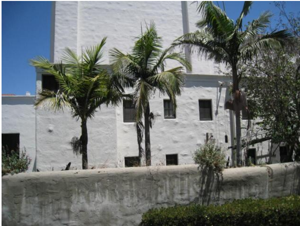
Plate 5. View from first level of parking garage of Green Room roof where added HVAC equipment will be hidden by high wall. Facing west.
