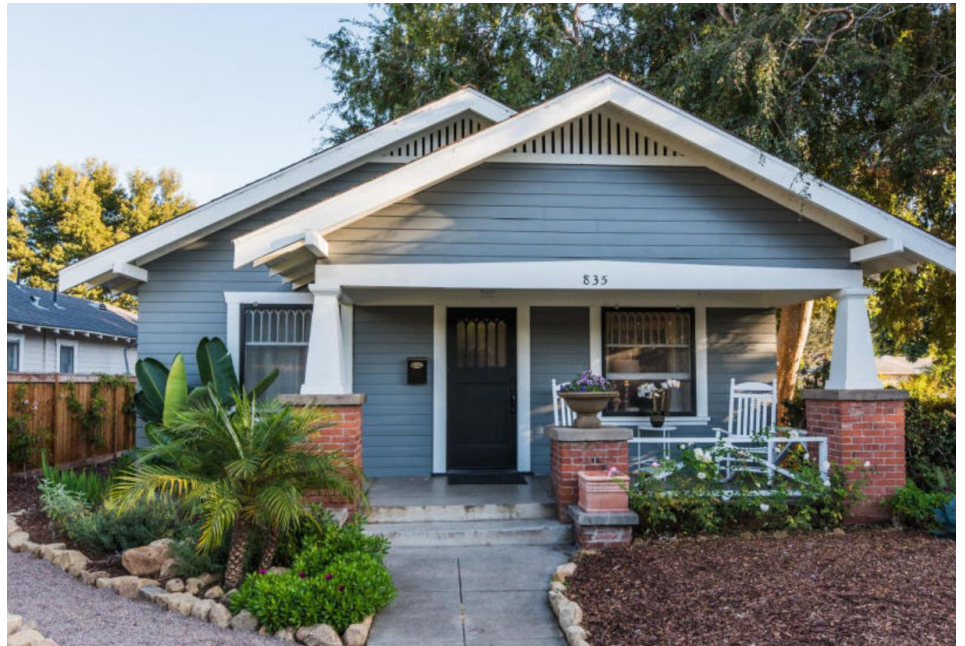
835 Alberta Avenue with low pitched, front facing gable roof over the porch with decorative vents under the open gables with tapered, square columns on massive brick piers and decorative design in the transoms and wood front door lights are character defining features of the Craftsman style. Photograph provided by applicant team April, 2024.
