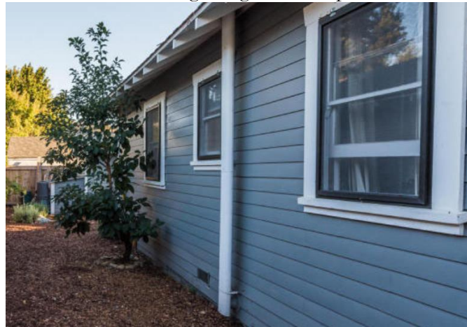
835 Alberta Avenue. Side elevation of the house showing original one-over-one windows with ogee lugs on the upper sash. Photos provided by applicant April 2024
