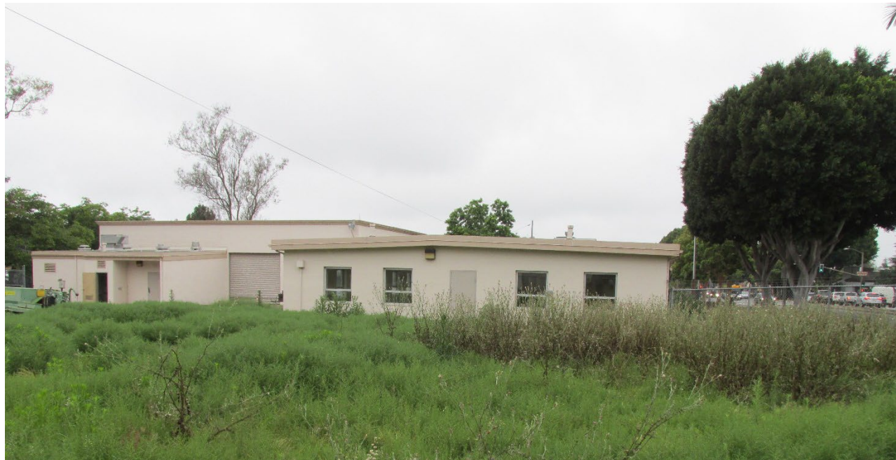
Figure 12. East elevation of Fremont Hall USAR Center showing Assembly Hall addition, looking west. (IMG_8349)
