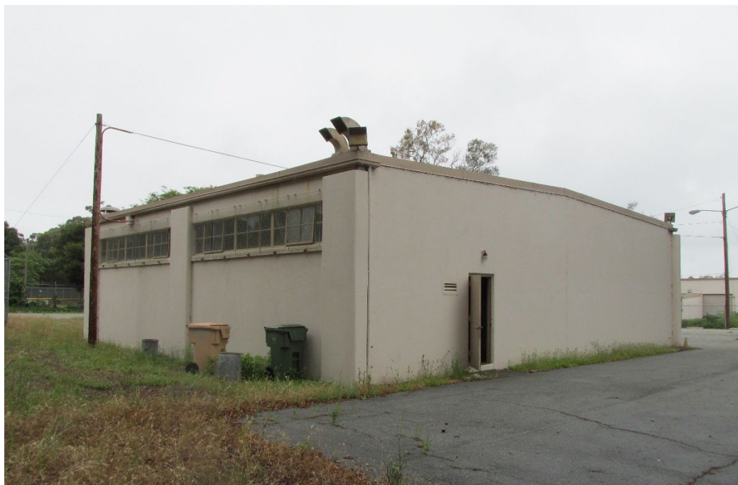
Figure 6. Organizational Maintenance Shop north and east elevations, looking southwest. (IMG_8341)
