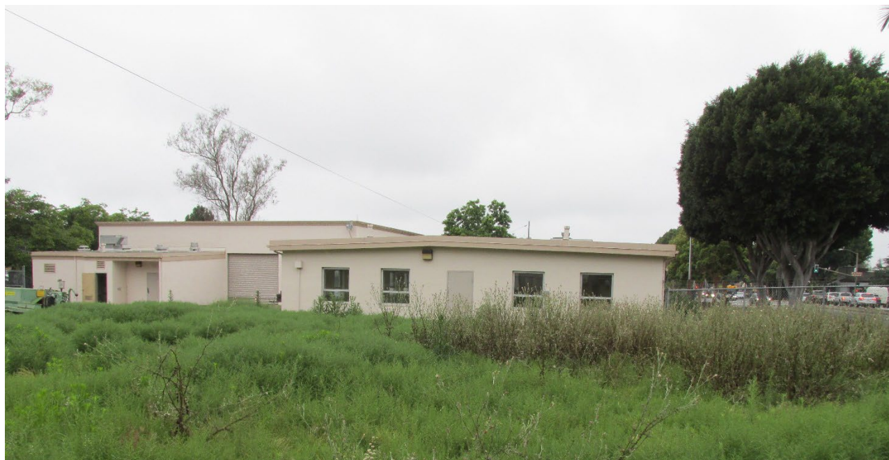
Figure 4. East elevation of Fremont Hall USAR Center showing Assembly Hall addition, looking west. (IMG_8349)
