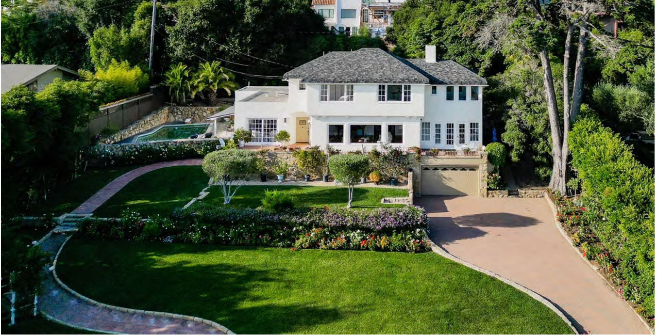
Figure 1, 1708 Paterna Road, looking north (APN 019-184-009) (Harrison Design and Interiors)
