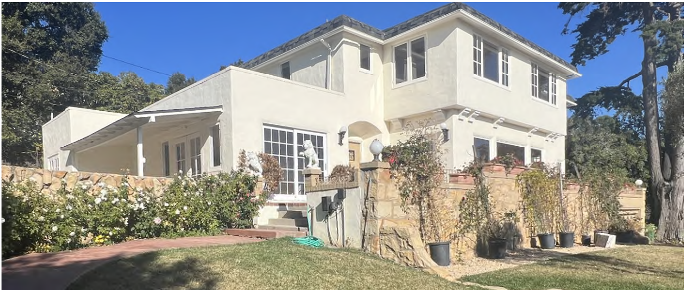
Figure 9, The west end of the south elevation and the west elevation with a detail of the sandstone retaining wall, looking northeast
