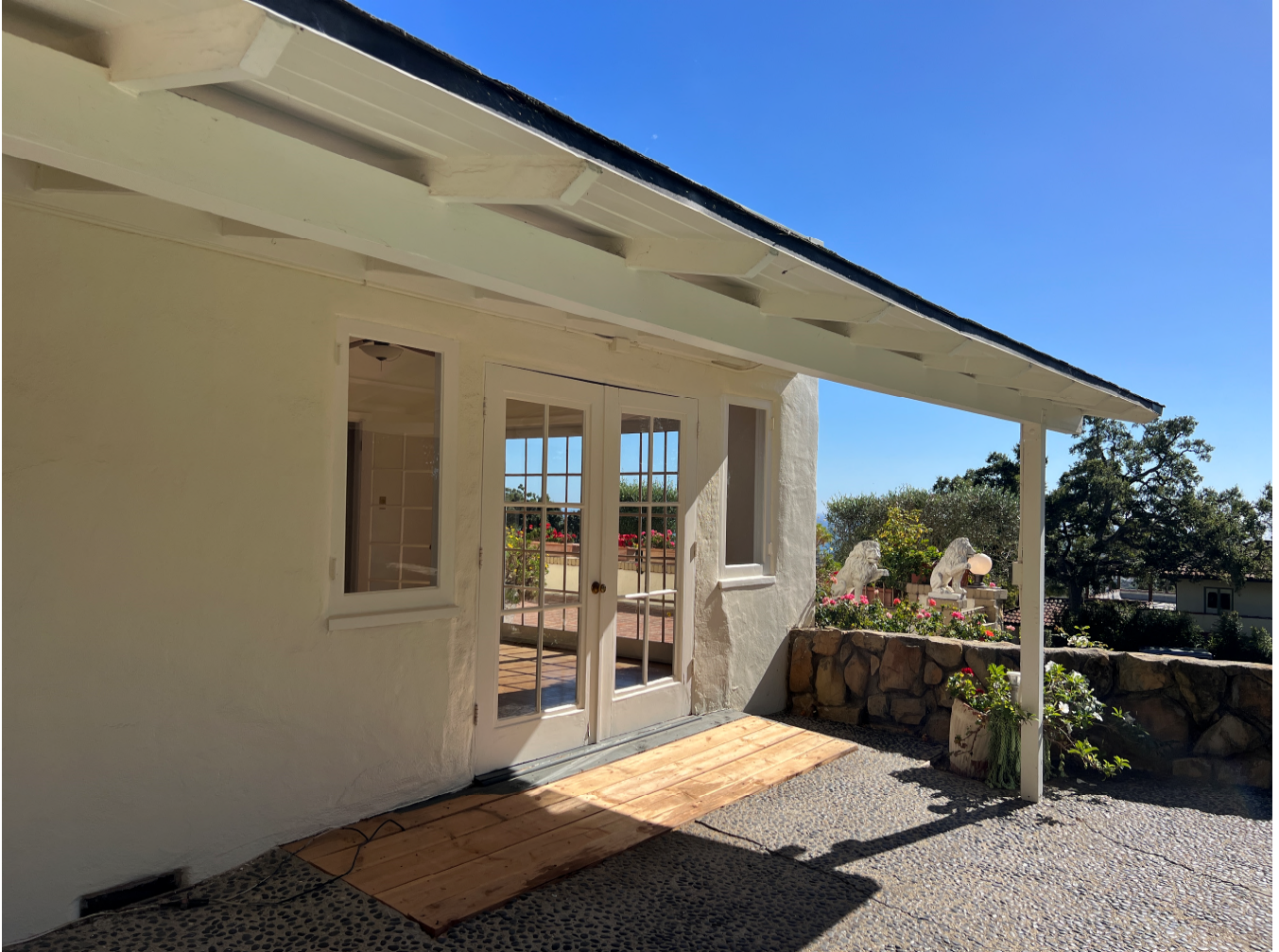
Figure 18, The west elevation with a detail of the porch, looking southeast
