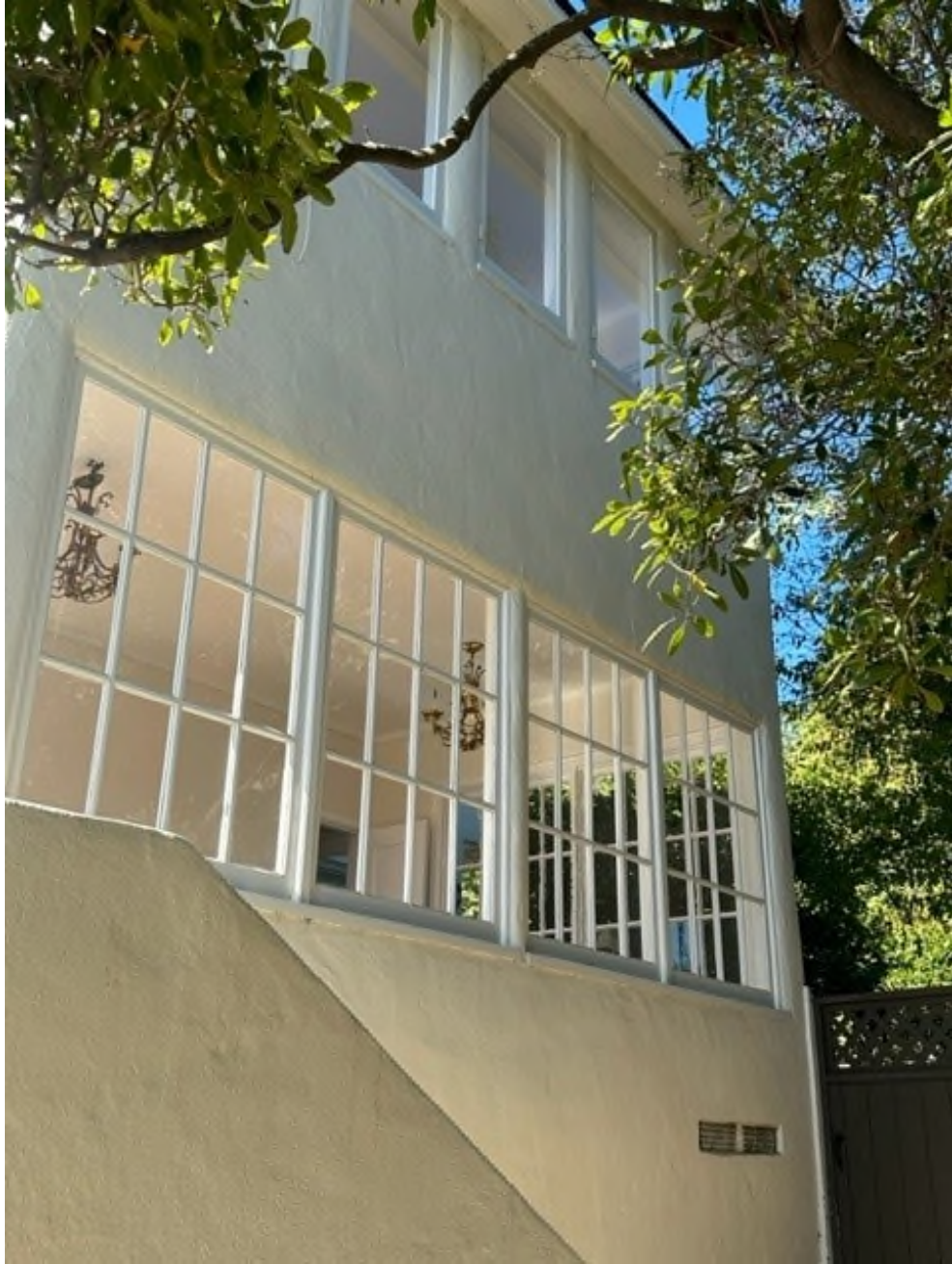
Figure 15, The east elevation, looking northwest
