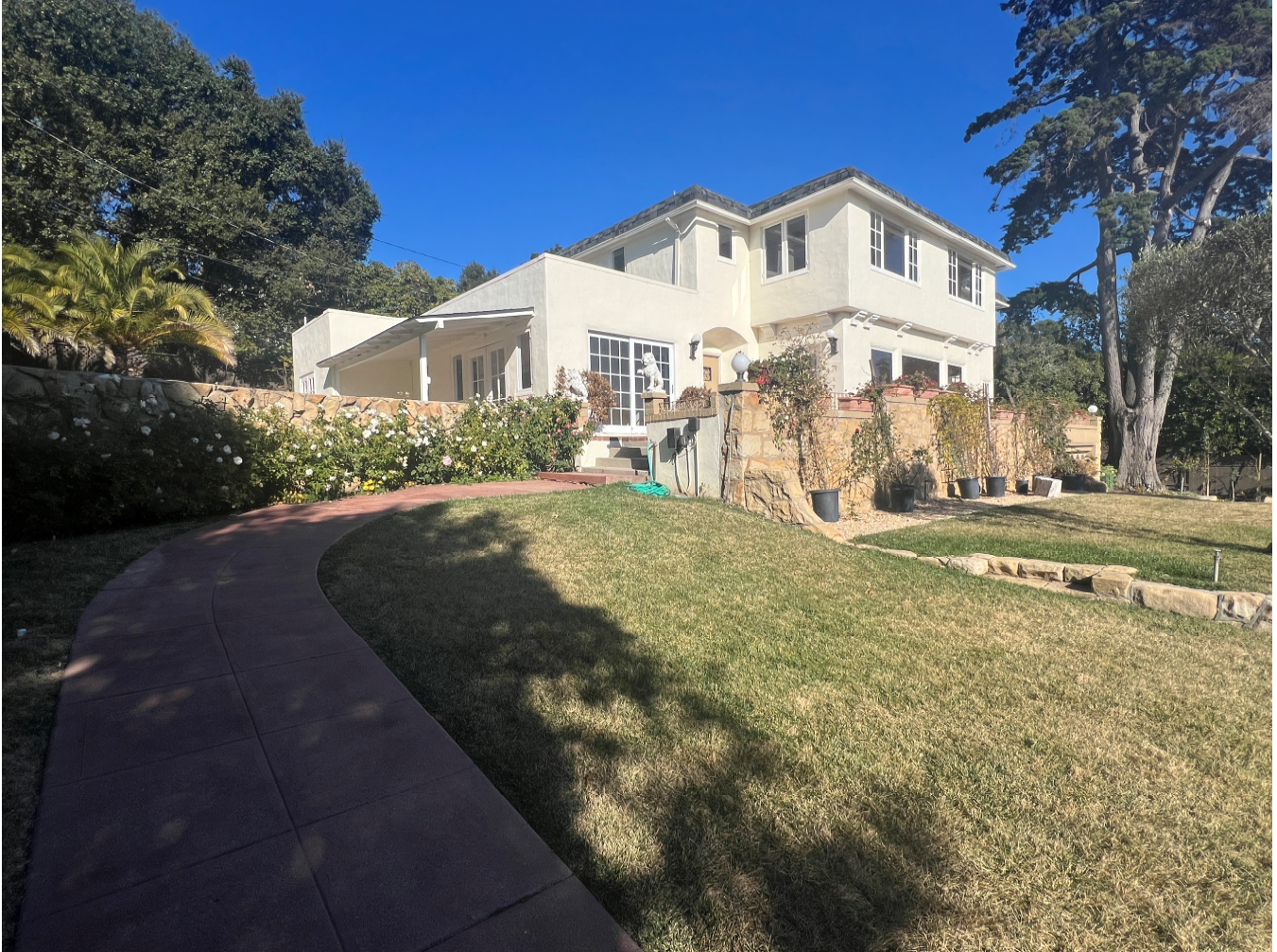
Figure 24, The concrete pathway leading from Paterna Road to the south elevation, looking northeast
