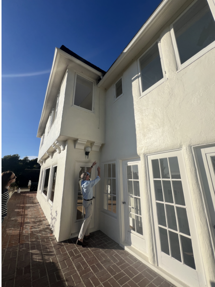
Figure 6, The central section of the south elevation, looking west
