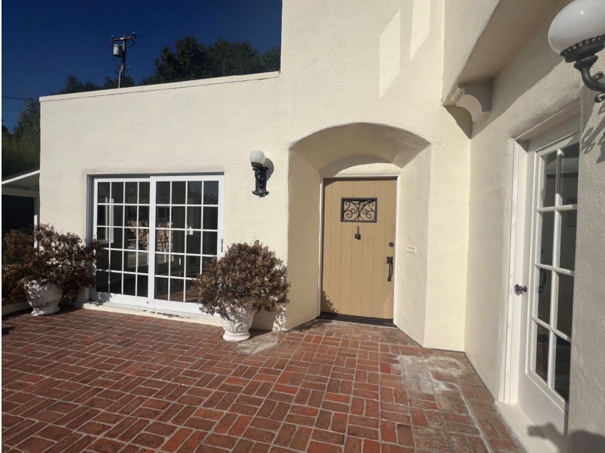
Figure 8, The west end of the south elevation, looking north
