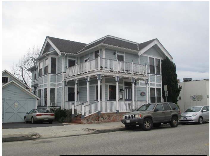
Above: 206 East Victoria Street, Bernasconi Residence at 206 East Victoria Street and its associated barn.
