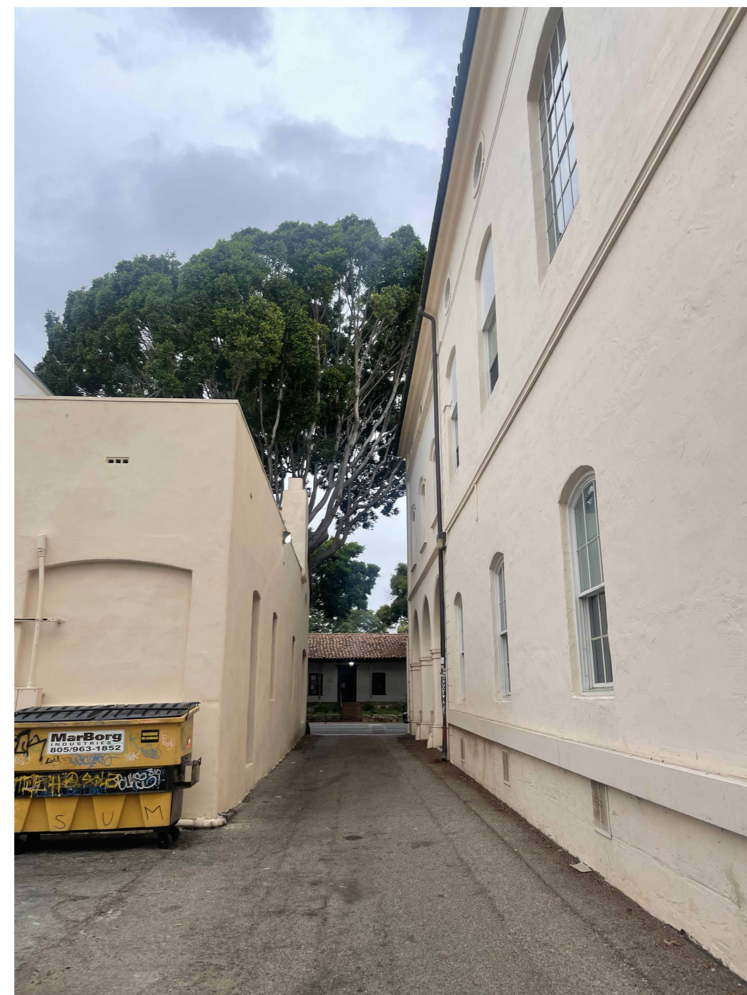
VIEW FROM ALLEY LOOKING TOWARDS CARRILLO ST
