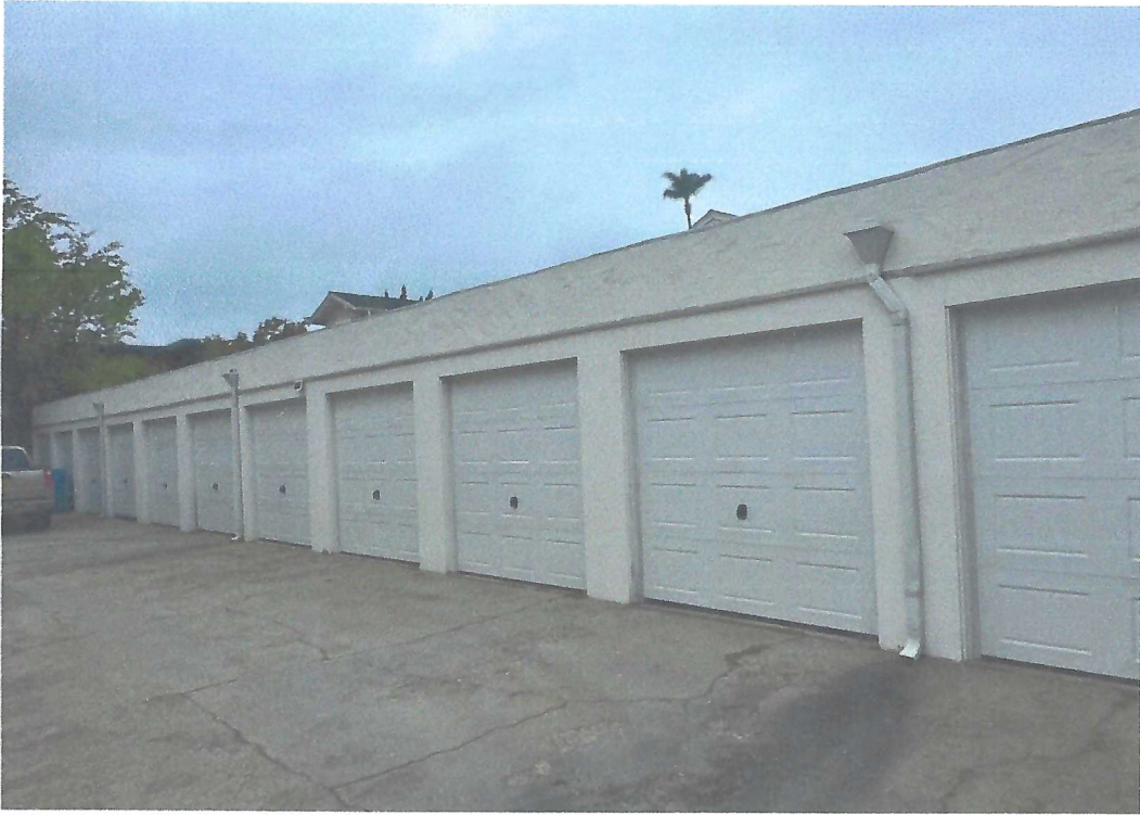
11 garages north side of property
