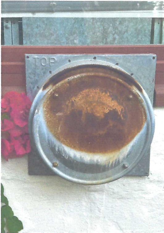
Existing gas vent
