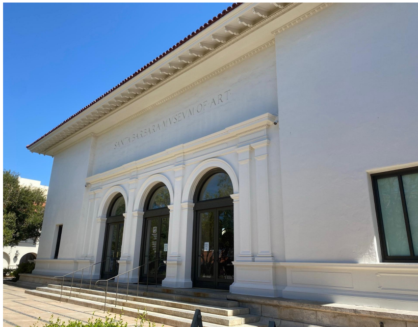
State Street (front) elevation, facing west
