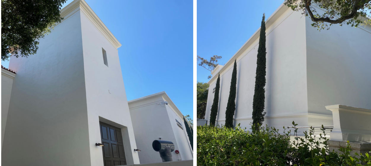
Northern elevation on East Anapamu Street
