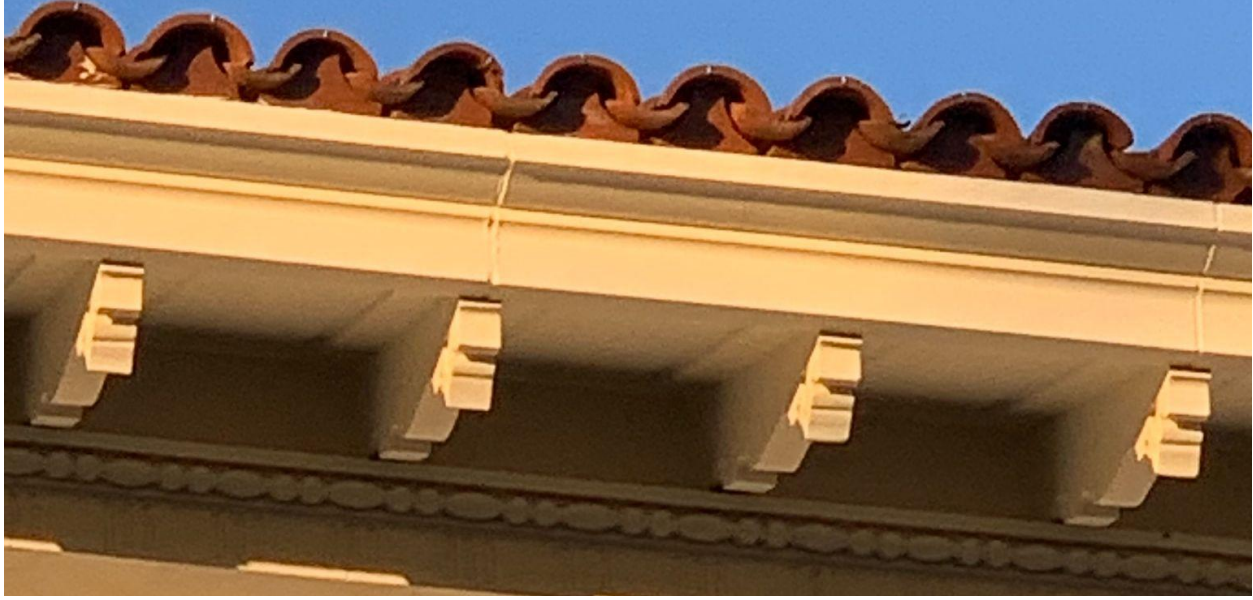
Cornice running around the facade underneath the terracotta tile barrels
