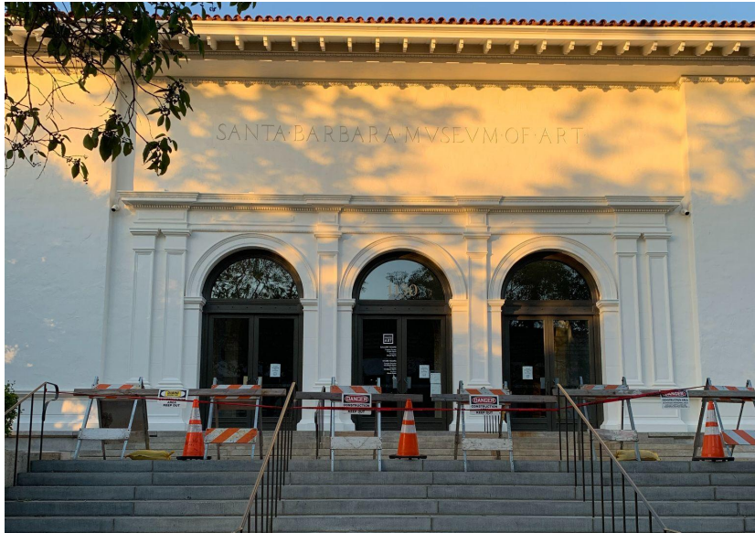
State Street (front/west) elevation
