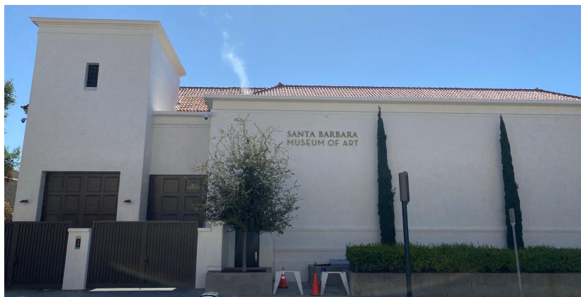
East Anapamu Street (side) elevation, facing north
