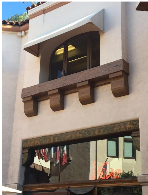
Above: Current view of the restaurant space behind the turtle pond, with the same ornately decorated lintel and heavy timber sill of the deeply recessed arched window of the second story as seen in 1930 photograph. Photo taken on September 25, 2017.
