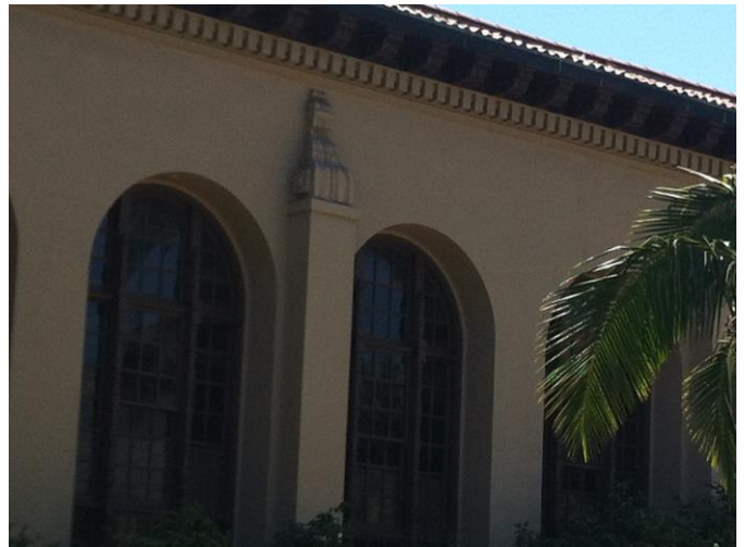
Intricately carved brackets over dentil molding and intricately carved wood window sashes of the Central Library. July, 2012.
