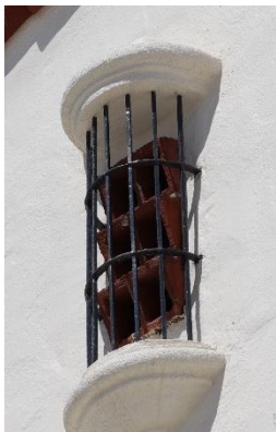
Figure 7 The iron rejas over the rain spouts from: Herics, Sebastian, 22 March 2021.
