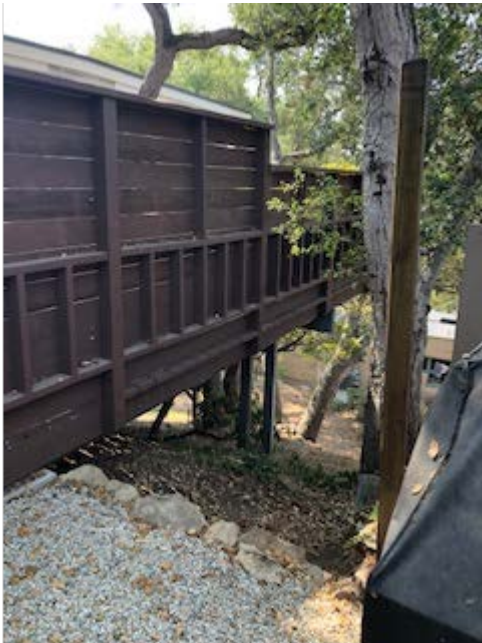
Photo of fence built on deck on alleged neighbor's property
