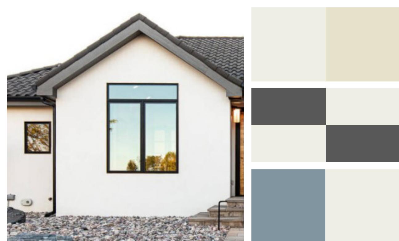
B.3 STUCCO Material: Stucco Plaster Finish, 7/8" Thick Color: White Dove (OC-17) Walls w/ Lancaster Whitewash (HC-174) Trim OR Peppercorn (SW-7674) Walls w/ White Dove (OC-17) Trim OR White Dove (OC-17) Walls w/ Peppercorn (SW-7674) Trim OR Poolhouse (SW 7603) Walls w/ White Dove (OC-17) Trim
