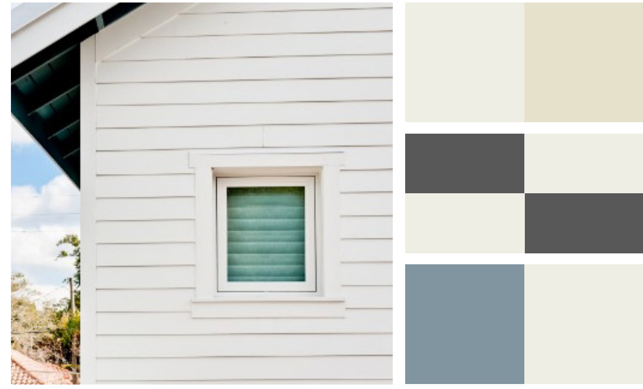
B.1 HORIZONTAL SIDING & TRIM Material: James Hardie Cementitious Siding Color: White Dove (OC-17) Walls w/ Lancaster Whitewash (HC-174) Trim OR Peppercorn (SW-7674) Walls w/ White Dove (OC-17) Trim OR White Dove (OC-17) Walls w/ Peppercorn (SW-7674) Trim OR Poolhouse (SW 7603) Walls w/ White Dove (OC-17) Trim
