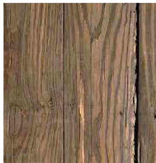
EXISTING/AS-BUILT FENCE ELEMENTS
