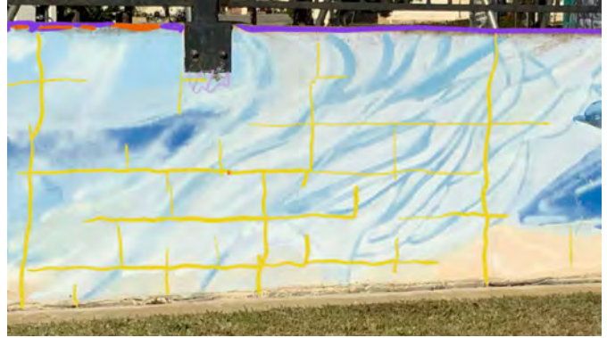
Figure 2. Example of the extensive cracking (drawn in yellow) in the shape of the CMUs found in Dolphins and Codex Cospi . This type and extent of cracking is what would make these murals extremely difficult to relocate without significant damage.
