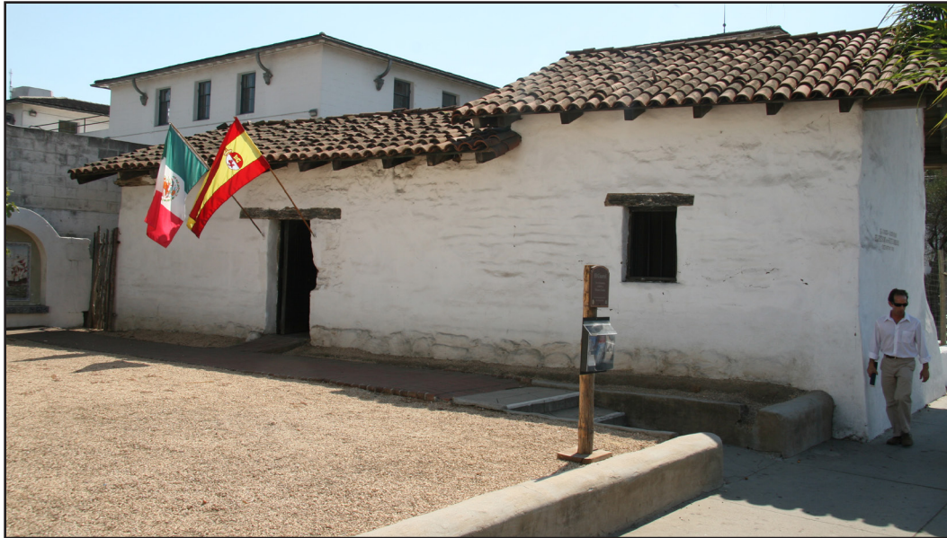
The thick walls of this adobe are covered with white plaster that gives it an undulating finish that hints at the adobe bricks underneath.
