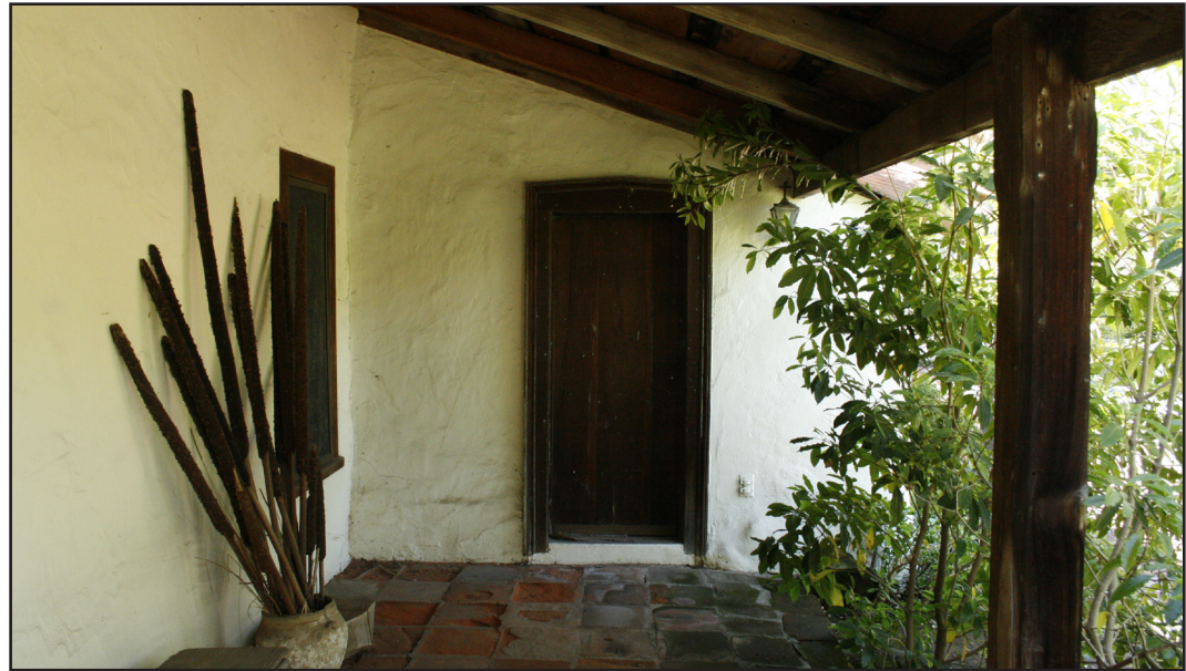
This adobe features porch posts made of thick wood timber. The door and window feature thick, unpainted trim.
