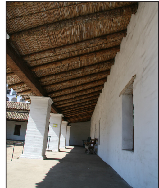
The long, narrow porch shows the underside of the roof featuring roof rafters that have reeds placed between them to provide support for the red clay roof tiles above.
