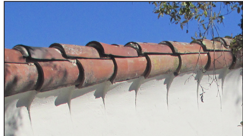
Side profile of clay tile along a gable end.
