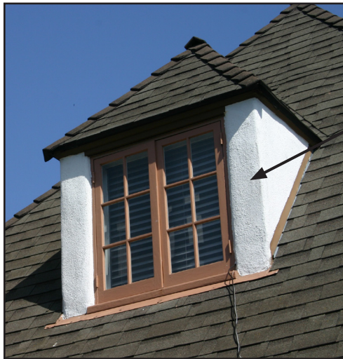
This dormer protrudes out of a composition roof that mimics the color and shape of original wood shingles.
