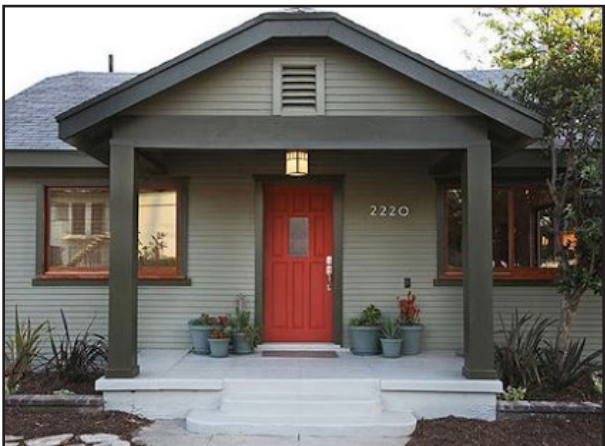
After: The wood sided bungalow after the stucco was removed and the character-defining wood siding restored. Photo from the eastsidela.com web site.
