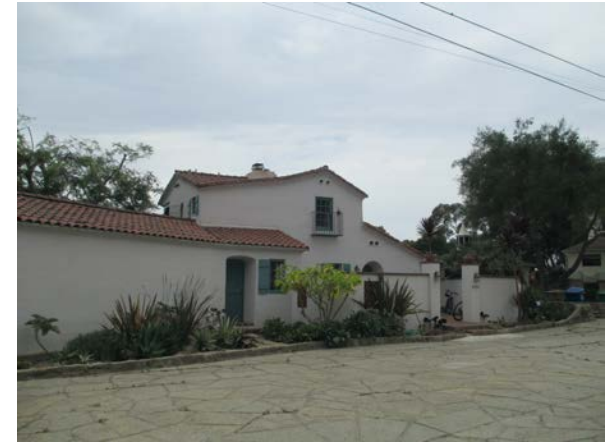
This Spanish Colonial Revival residence features the deeply recessed openings along smooth stucco walls that are unique to the Spanish Colonial Revival style.
