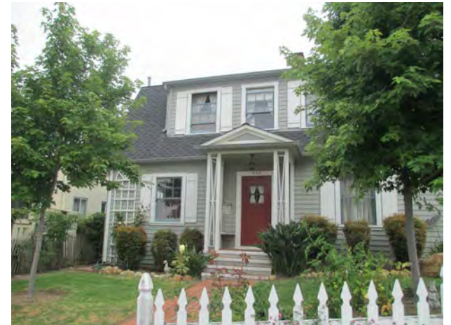
The 1922 American Colonial Revival house on Montgomery Street is typical of the eclectic array of houses designed in period revival styles in the historic district.
