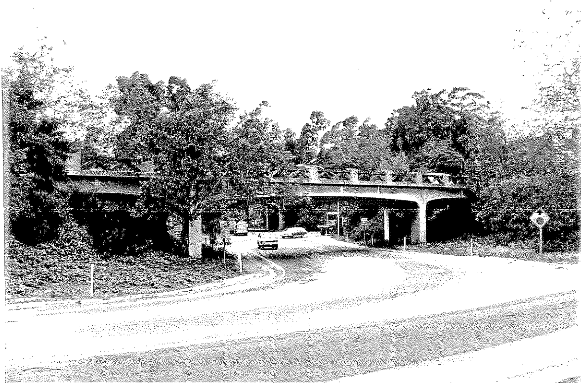
PHOTO 18: Hot Springs Road/Cabrillo Blvd. interchange: Looking south to northbound bridge
