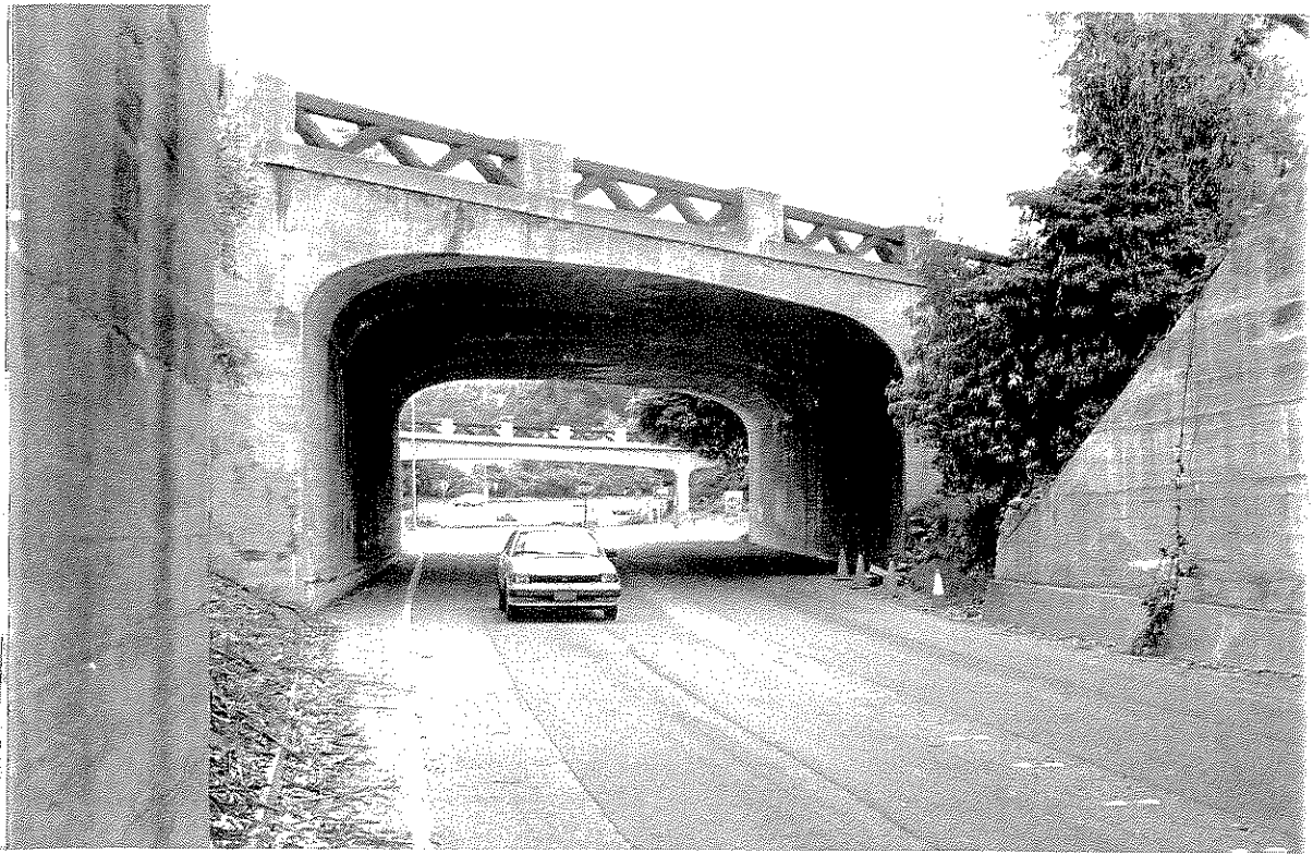
PHOTO 17: Hot Springs Road/Cabrillo Blvd. interchange: Looking toward southbound bridge
