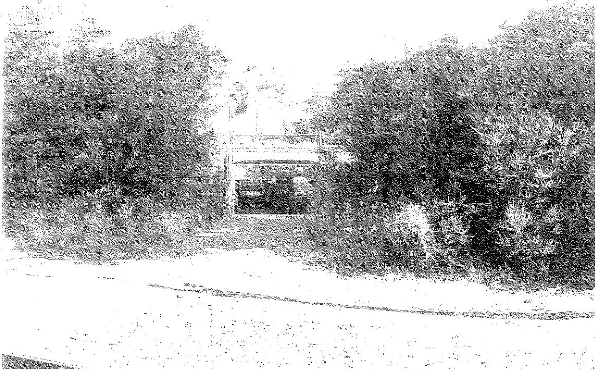
PHOTO 25: Butterfly Lane Pedestrian Undercrossing
