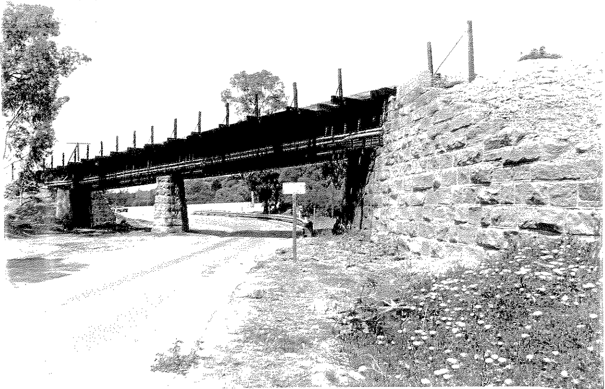
PHOTO 23: Los Patos Way Railroad Bridge
