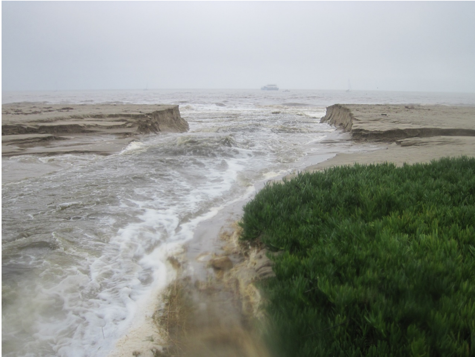
Photo - 8 Beach Berm Breach (East Beach) – 1100 E. Cabrillo Blvd
