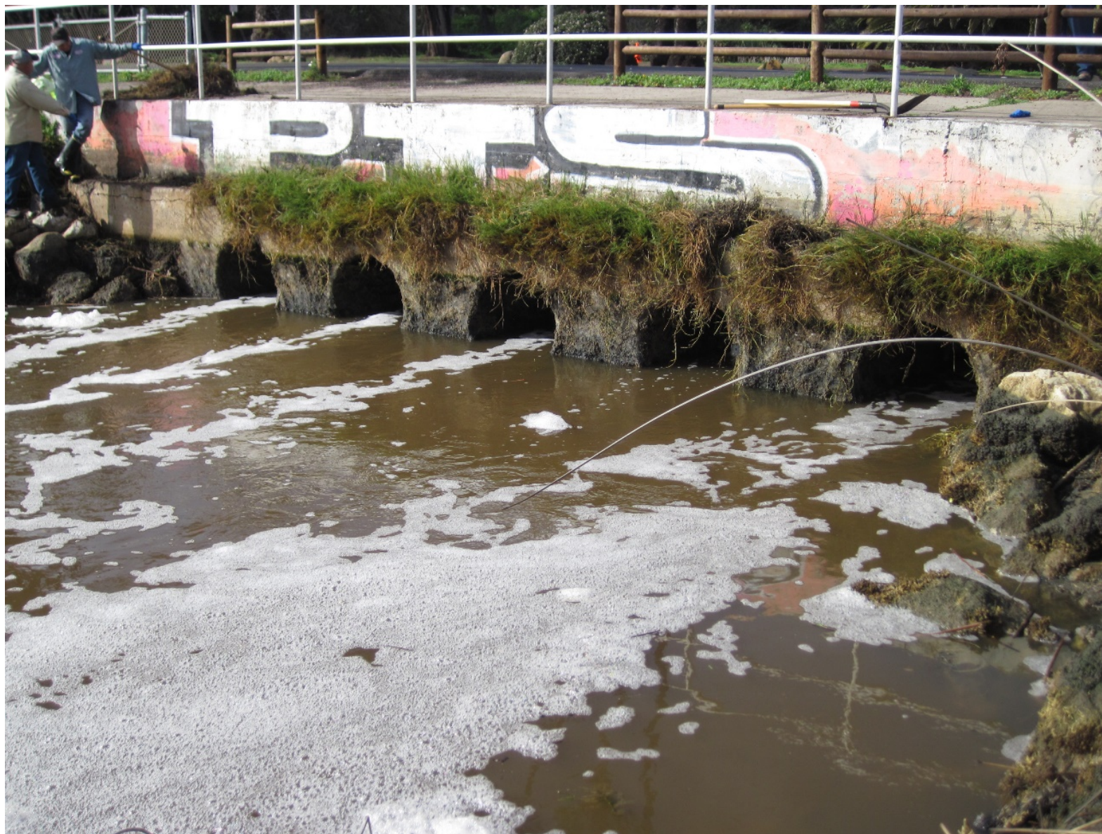
Photo 4 - Culvert Outflow Under South Side of E. Cabrillo Blvd – 1110 E. Cabrillo Blvd
