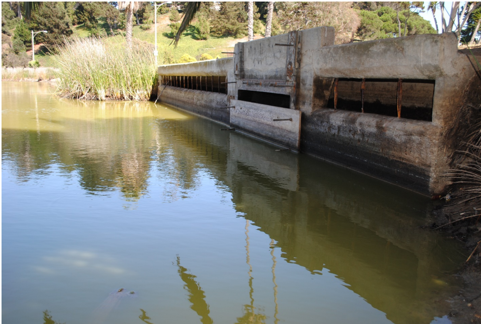
Photo - 6 Concrete Weir/Dam North Side of E. Cabrillo Blvd (Bird Refuge Lagoon) – 1100 E. Cabrillo Blvd
