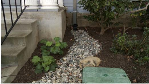
The old lawn sprinkler system was easily retrofitted to a low flow, low pressure drip system and “once this landscape is established, it is estimated that it will reduce the water consumption by 75-85%,” said Daniel Wilson. Additionally, the maintenance required is expected to drop by 99%! The old garden required mowing once a week, quarterly fertilizing, and weekly hauling of green waste. Now it will only require quarterly pruning for shaping, no power tools needed.
