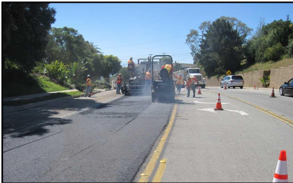
The crews place the hot asphalt concrete and compact with roller.
