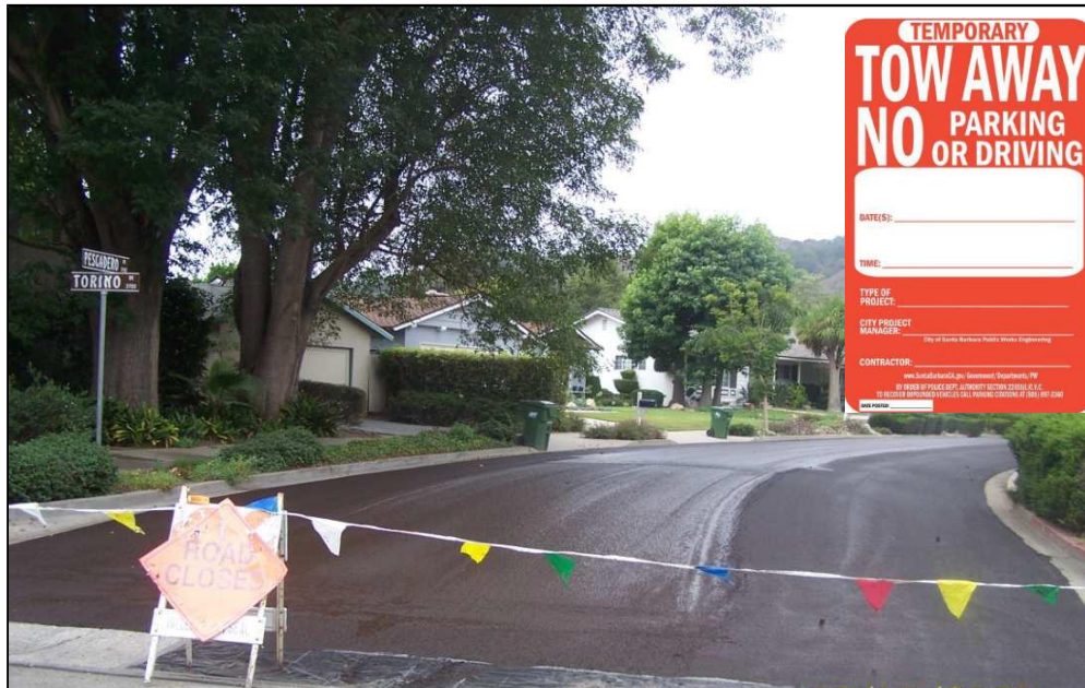
After the slurry seal is applied, the road is closed to traffic, and no parking is allowed.
