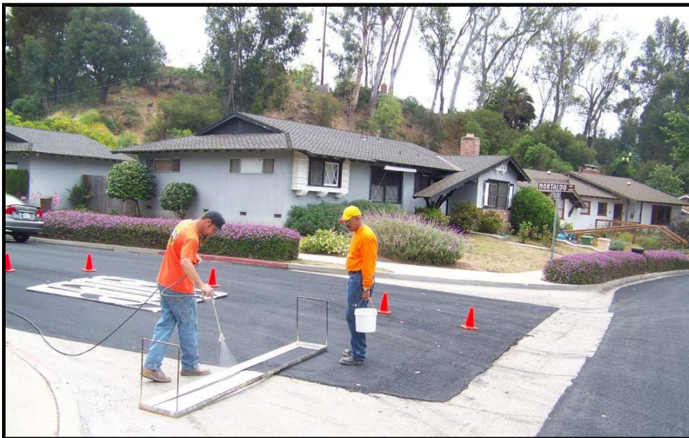
As a last step, the three coats of traffic stripe painting are applied.
