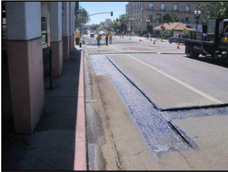
The crew "tack coats" the edges of the existing asphalt concrete so that it bonds with the new asphalt.
