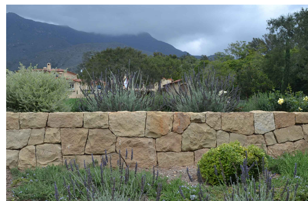
Fitted Santa Barbara Sandstone Wall
