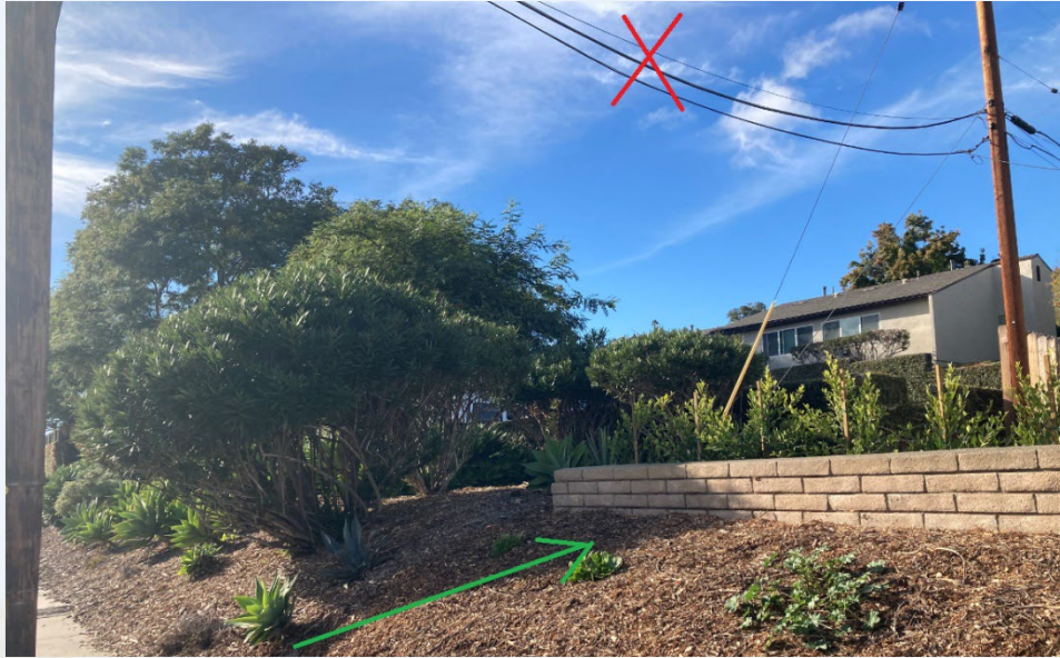
Example Underground Trenching Required Within Utility Easements - Softscape
