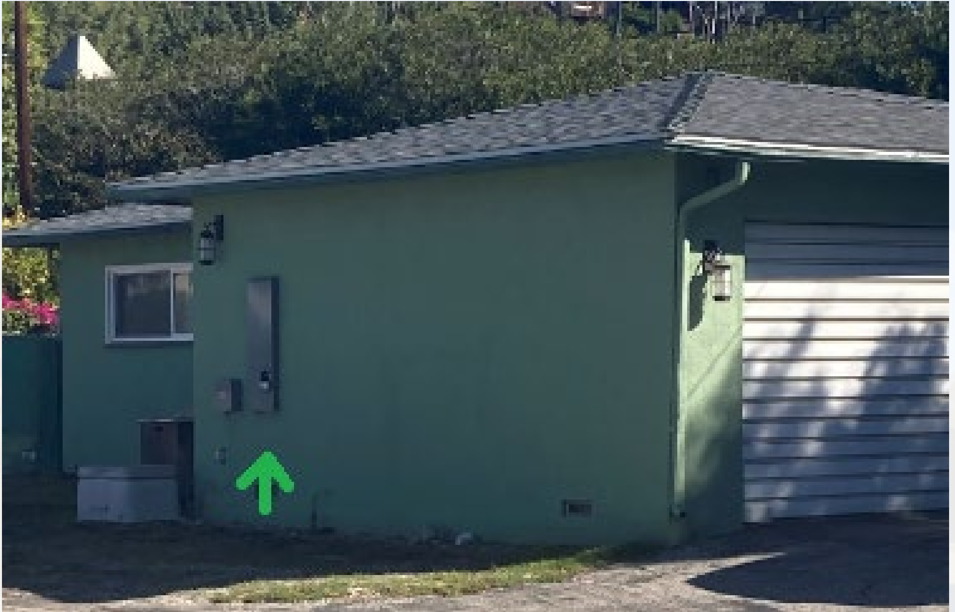
Example Underground Electric Meter – All Properties Within the Boundary on North Side of Cliff Drive Must Convert from Overhead to Underground
