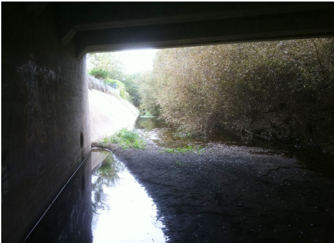
Photo 10: Underneath Gutierrez Street Bridge, upstream view
