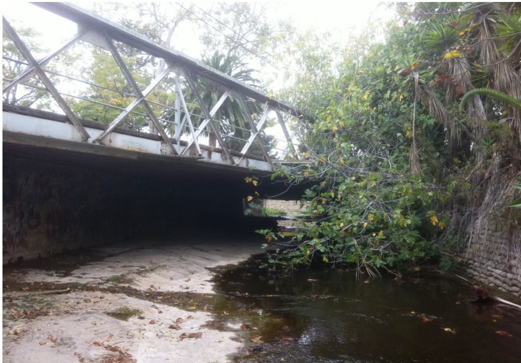
Photo 16: Immediately downstream of Chapala/Yanonali Street Bridge, upstream view (upper end of tidal influence)
