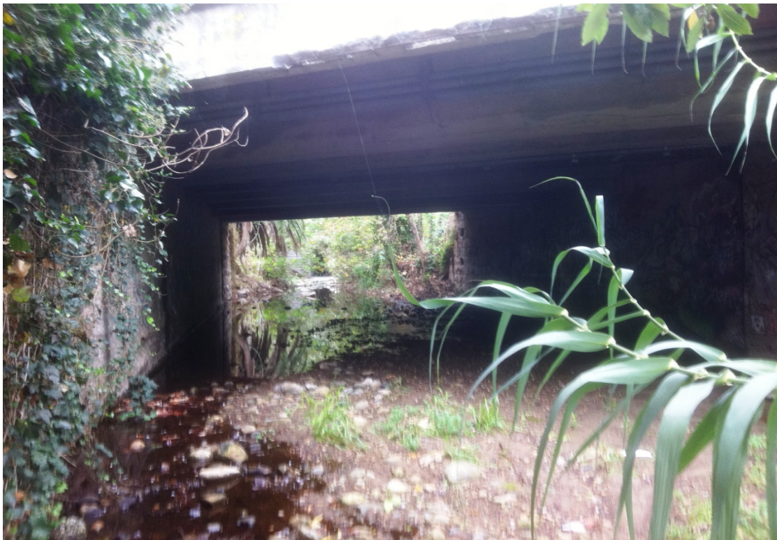
Photo 6: Immediately downstream of Cota Street Bridge, upstream view
