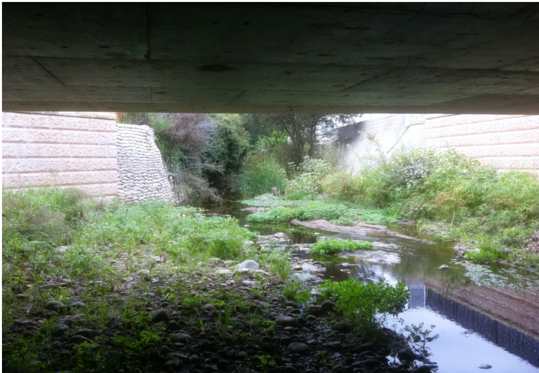
Photo 8: Underneath Haley Street Bridge, upstream view
