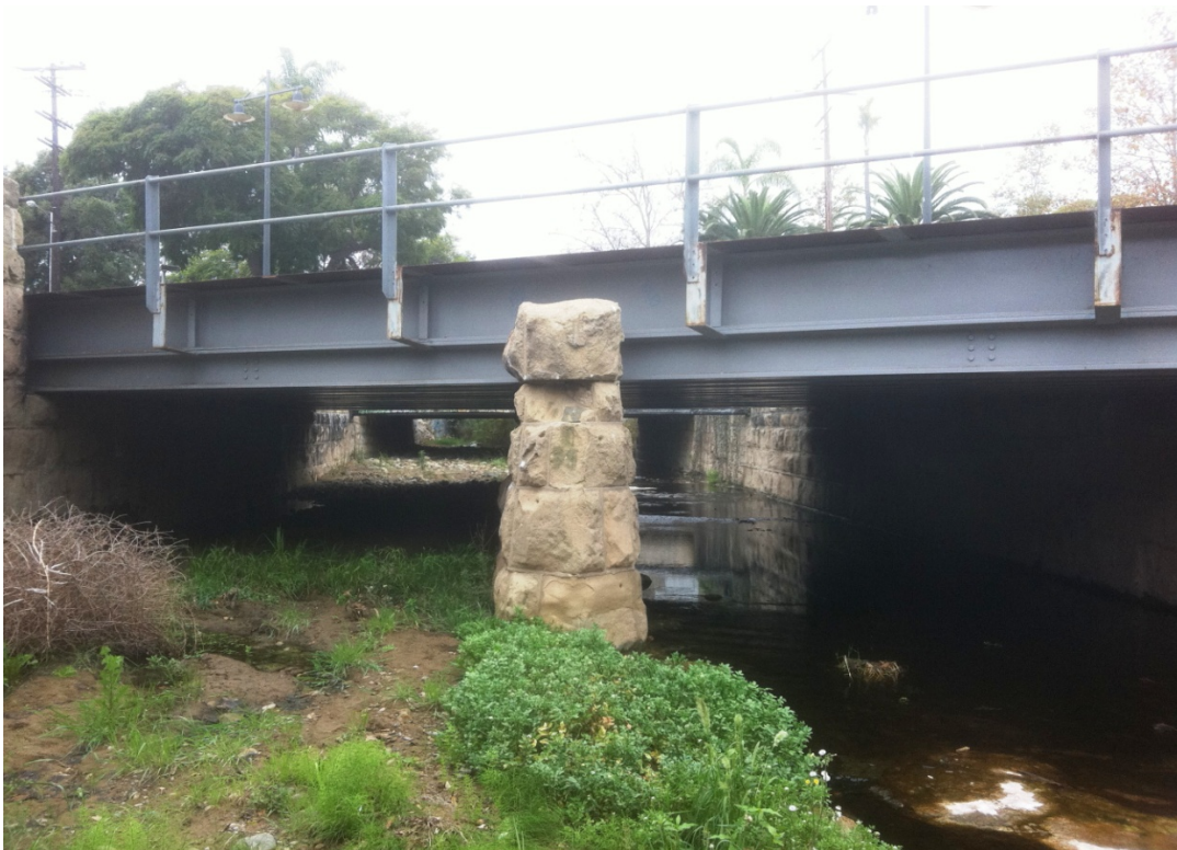
Photo 14: Immediately downstream of Railroad Bridge, upstream view
