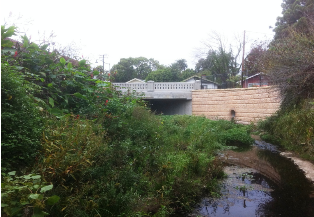
Photo 9: Immediately downstream of Haley Street Bridge, upstream view
