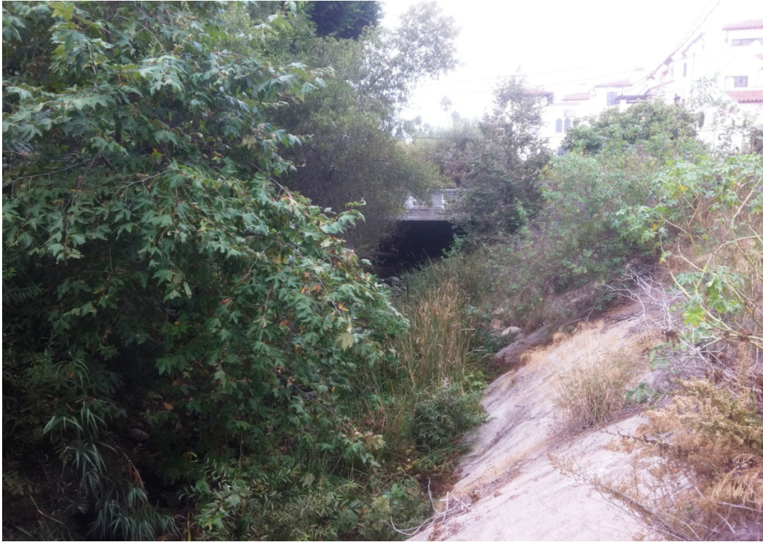
Photo 11: Immediately downstream of Gutierrez Street Bridge, upstream view
