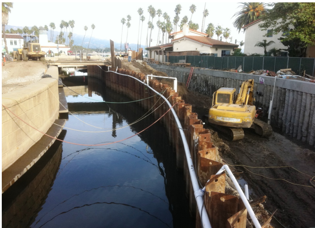
Photo 18: Downstream end of Project reach, Between Mason and State Street Bridges, downstream view (construction of Reach 1A, phase 1, Santa Barbara County)
