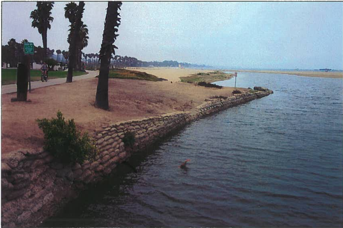
Photograph No. 3. View of eastern banks of lagoon near the bike path. Note concrete sandbag walls and eroded slopes.
