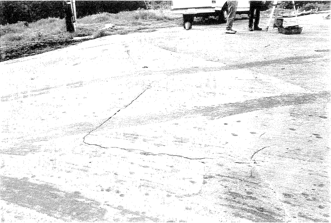
Photo 3 Pavement cracking Conejo Road Slide Mass A near survey monitoring point 5043, 1/13/05.
