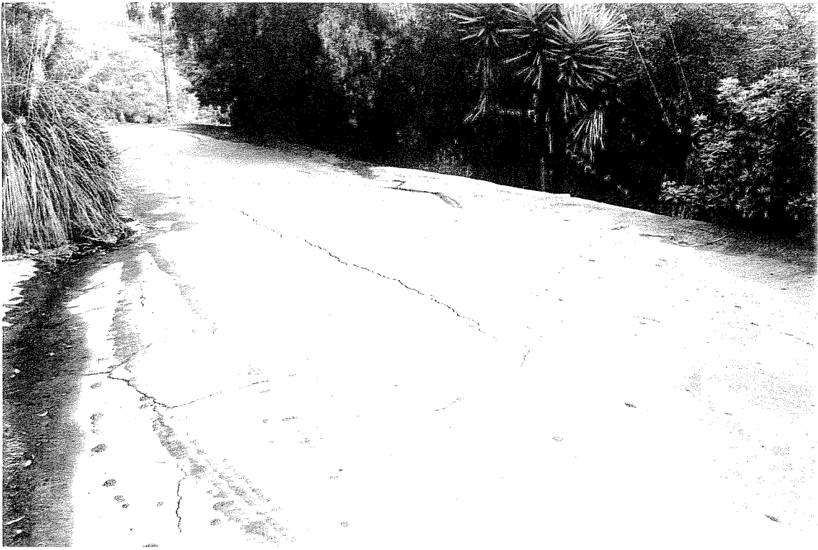
Photo 9 Pavement cracks near 428 Conejo Road, 1/13/05.
