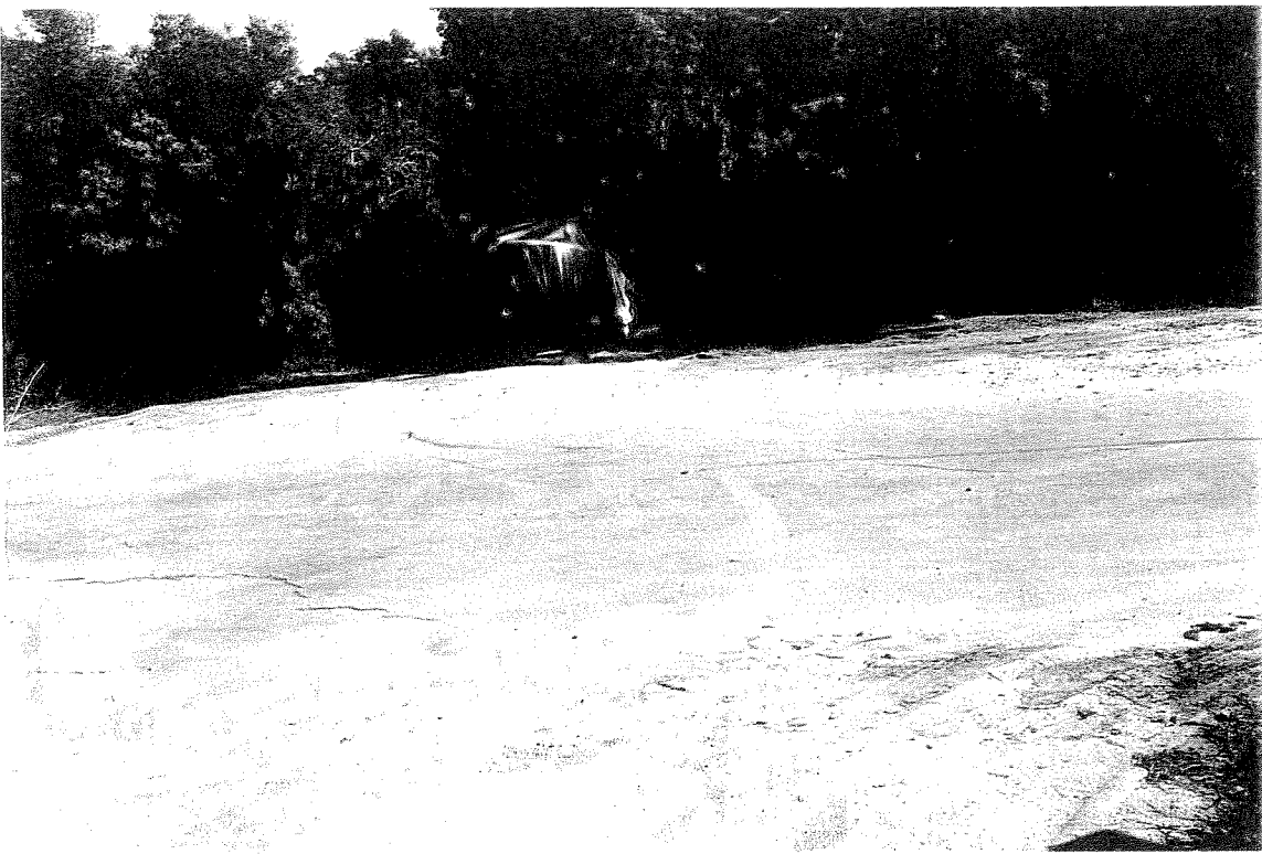
Photo 5 Pavement cracks Conejo Road slide Mass A near the Conejo Road / Conejo Lane intersection, 2/1/05.
