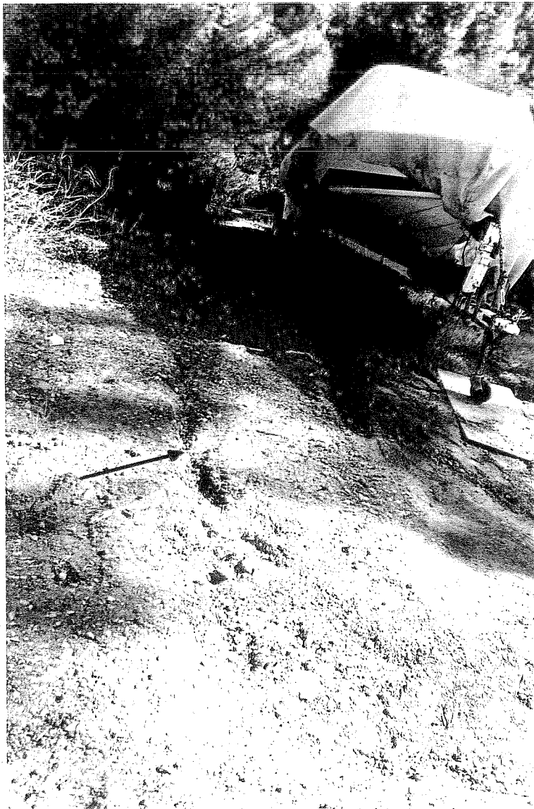
Photo 5 Pavement cracks Conejo Road slide Mass A near the Conejo Road / Conejo Lane intersection, 2/1/05.
