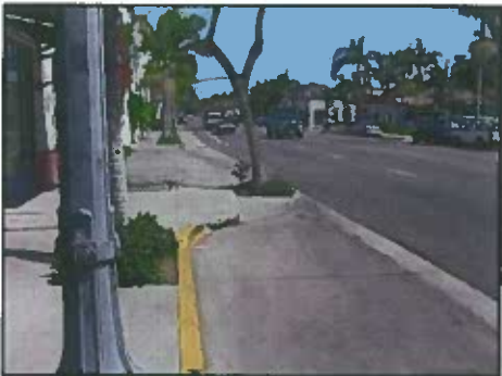
Curb extensions can shorten crossing distance.
