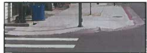
Two ramps is the preferred design.
