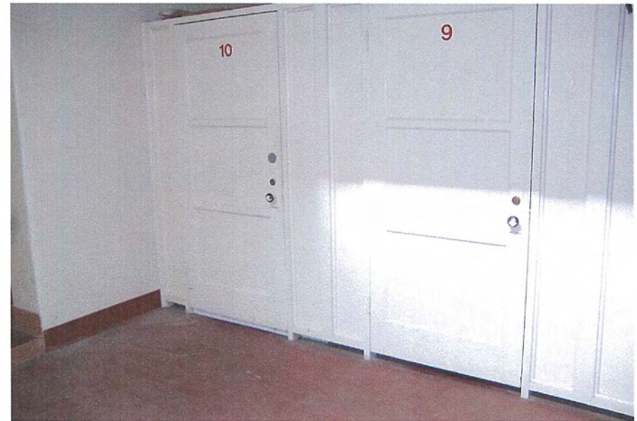
Building - Photo # 4 Storage cubicles do not have compliant hardware, knobs require tight grasping and twisting of the wrist.
