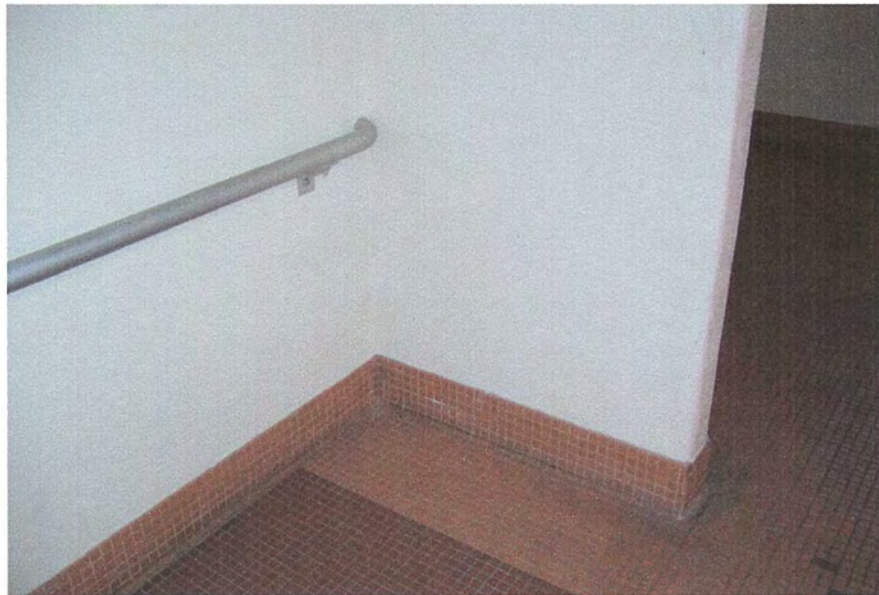
Building - Photo # 3 Handrail dead-ends on wall.
