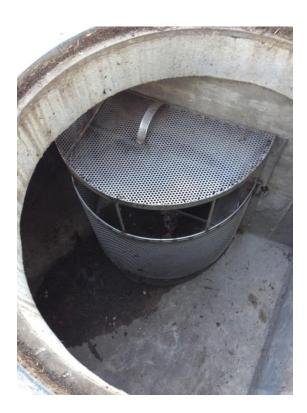
Figure 1. Photo of trash excluder. Photo Courtesy of the City of Ventura.
