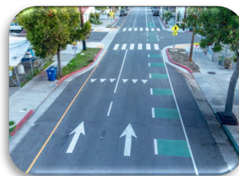
Green Conflict Striping
