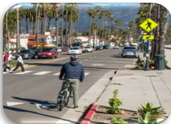
Pedestrian Activated Rectangle Rapid Flashing Beacons
